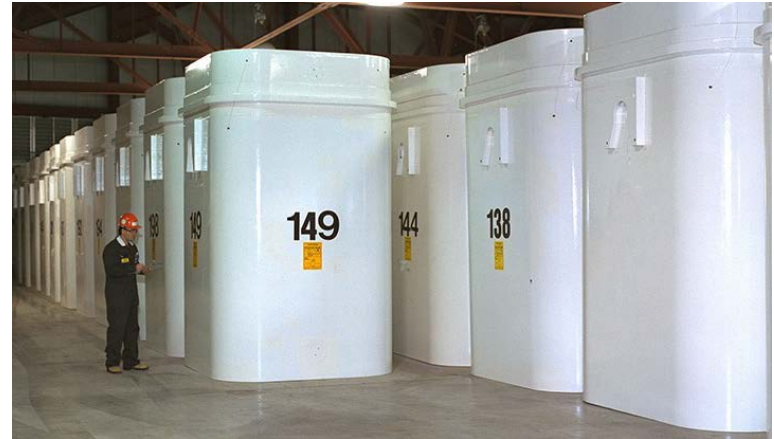
Used fuel Dry Storage Containers, Pickering Waste Management Facility.
