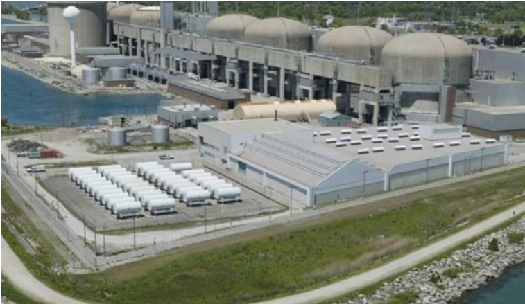
Pickering Waste Management Facility Phase I with retube component storage area (left) and used fuel dry storage buildings (right).
