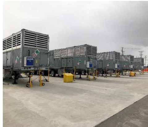
Figure 2: EME Phase 2 fans for ensuring control of Hydrogen in the Irradiated Fuel Bays (left); and five EME Phase 2 generators ready for deployment (right)
