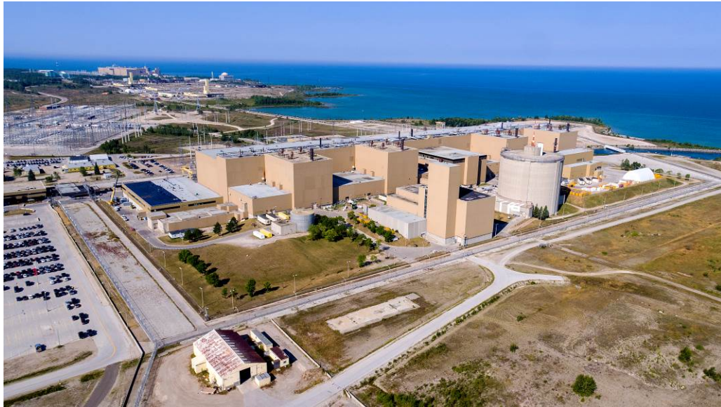
Figure 1: Aerial view of Bruce A
