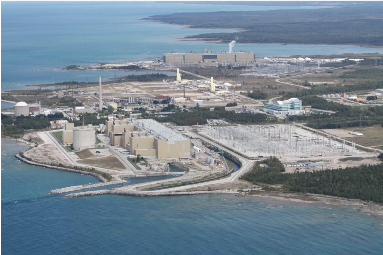
Figure 1.2: Aerial view showing Bruce B in foreground and Bruce A in background
