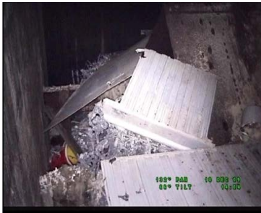
Intermediate level waste inside a legacy silo
