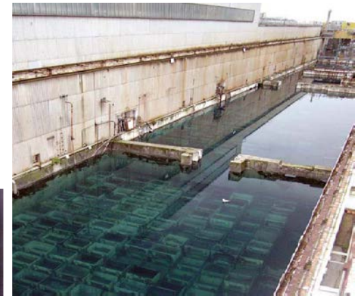
Irradiated fuel and sludge in a legacy pond
