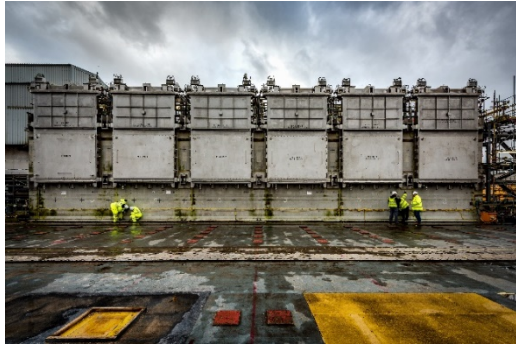
Pile Fuel Cladding Silo
