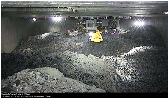
Beginning of FED removal
