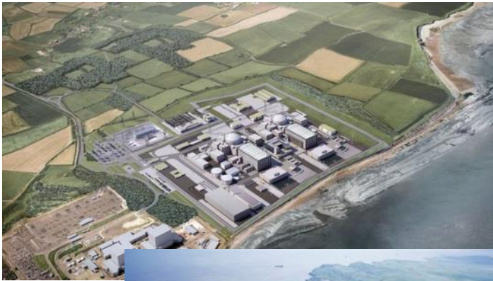
Hinkley Point C, copyright of EDF Energy
