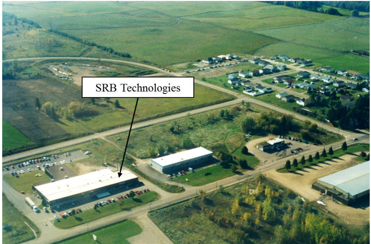
Figure 8-1: Aerial view of the SRBT facility
