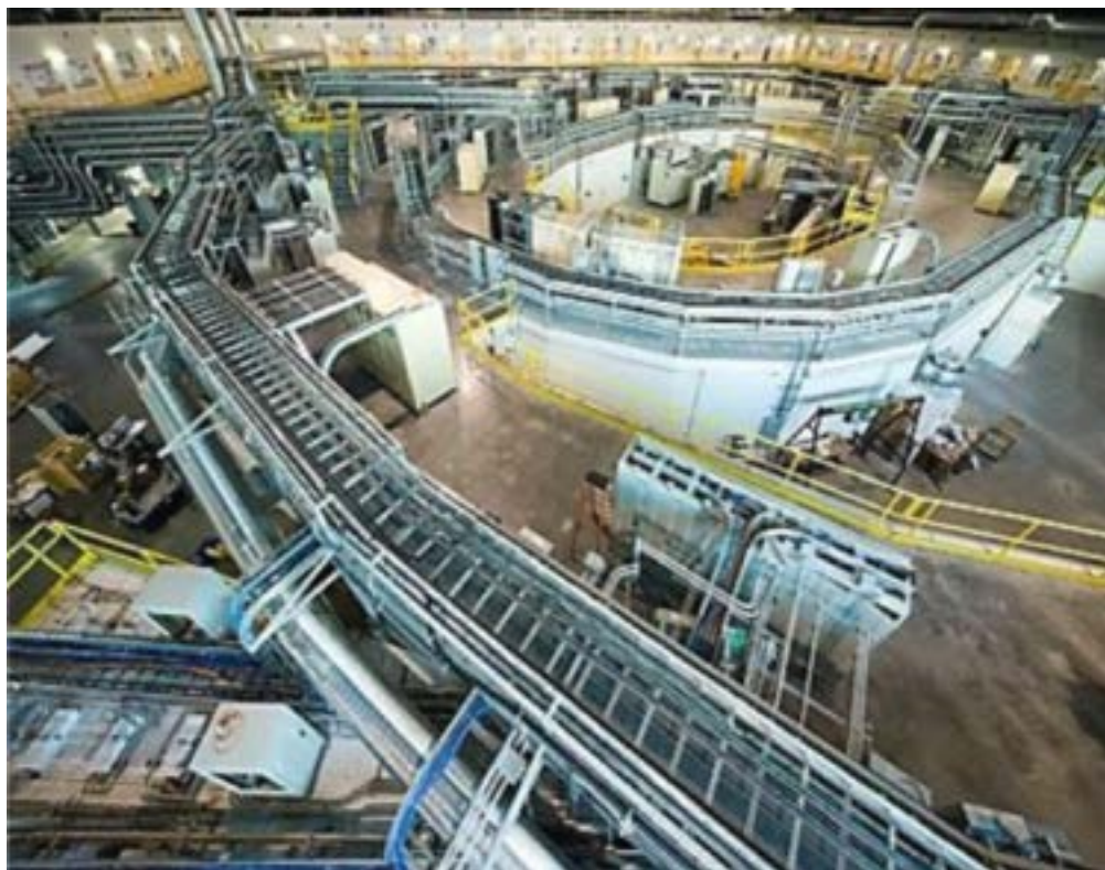
Figure 16-2: Inside view of the Canadian Light Source Inc. facility
