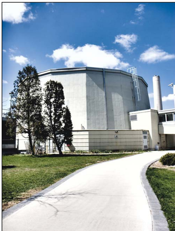
Figure 12-2: Ground-level view of the McMaster Nuclear Reactor facility
