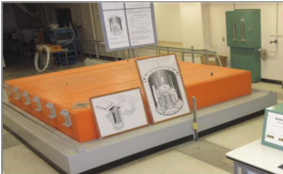
Figure 13-5: Top of the University of Alberta SLOWPOKE-2 reactor, covered with concrete blocks
