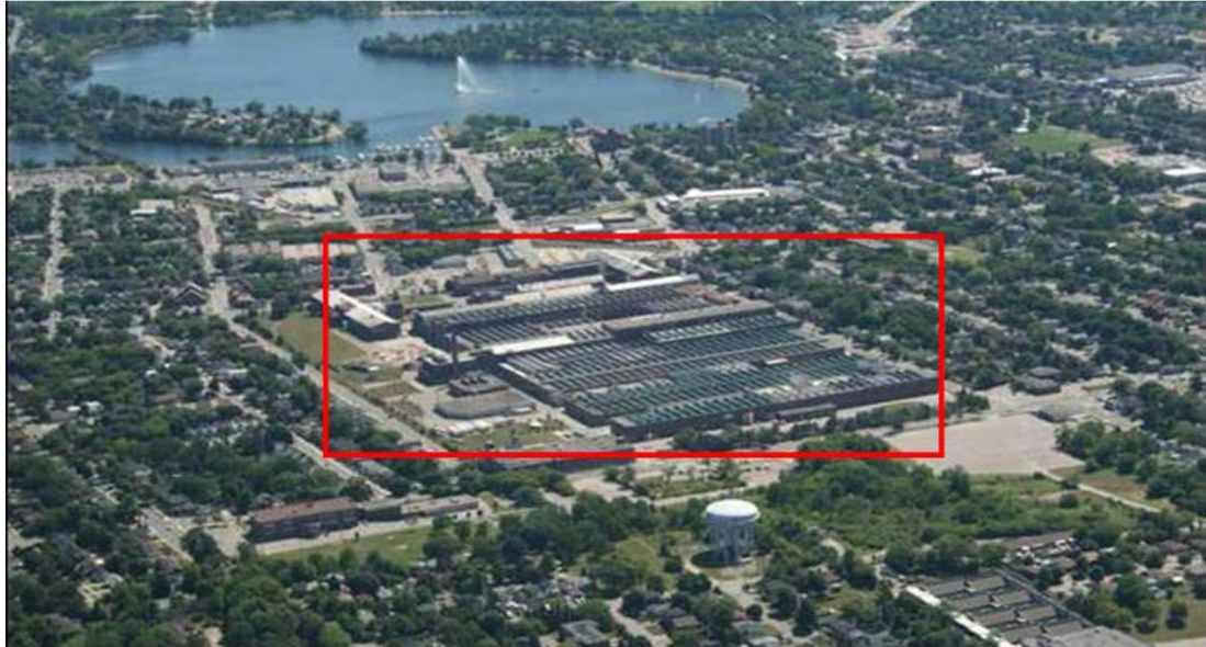
Figure 6-2: Aerial view of the GEH-C Peterborough facility
