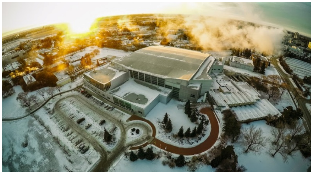
Figure 16-1: Aerial view of Canadian Light Source Inc. facility
