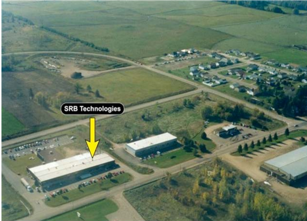
Figure 8-1: Aerial view of the SRBT facility
