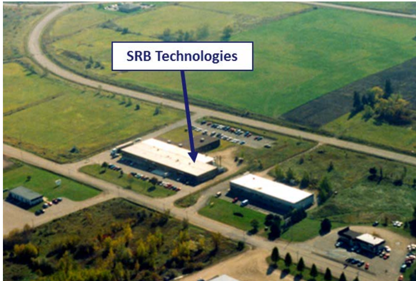
Figure 8-1: Aerial view of the SRBT facility
