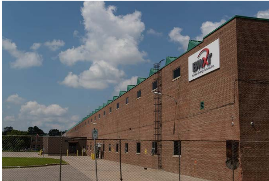
Figure 6-2: Side view of the BWXT Peterborough facility
