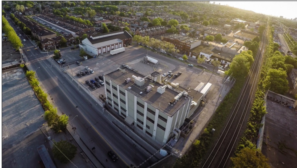
Figure 6-1: Aerial view of the BWXT Toronto facility
