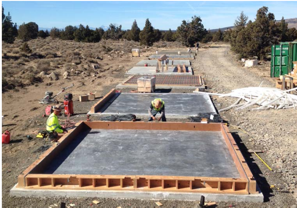
Figure 2-3: Mud Mat Construction
