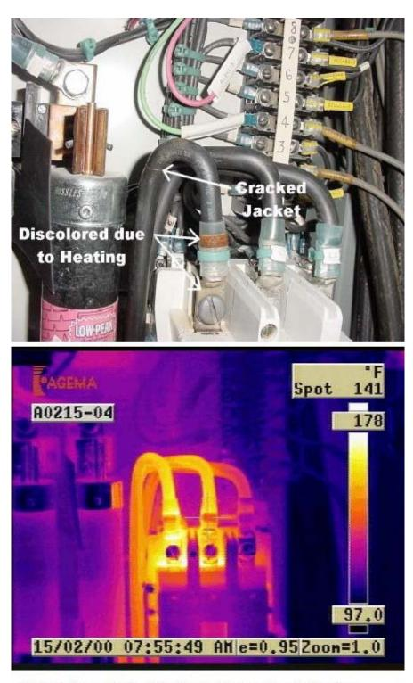
First photo shows cable degradation from local hot spots. Second photo shows thermograph of same cables. (Photo courtesy of Cooper Nuclear Station)
