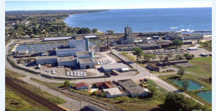
Port Hope Conversion Facility
