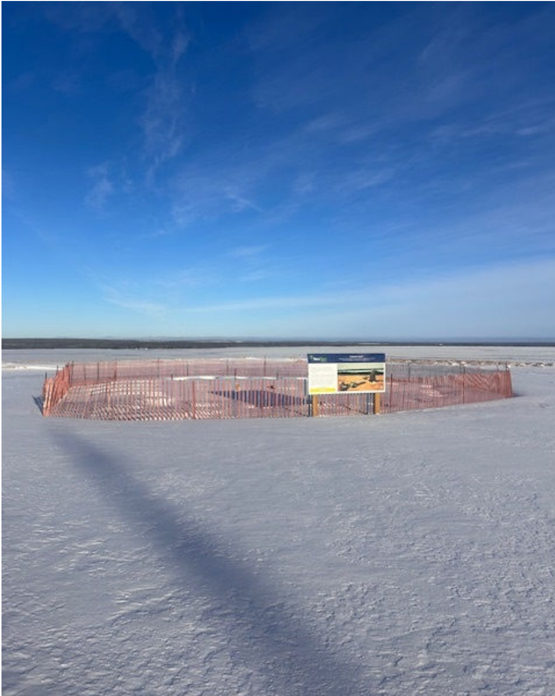
East drill pad -Exhaust shaft November 19, 2024
