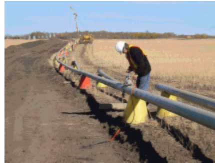
Image 6: NDT Pipeline inspection, using industrial radiography equipment
