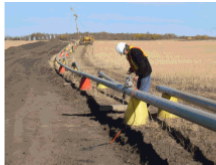
Image 6: NDT Pipeline inspection, using industrial radiography equipment
