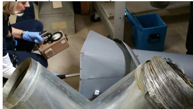
Figure 8: Checking for contamination during an inspection (Source: CNSC)
