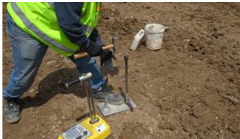
Figure 62: Portable gauge being used at a construction site (Source: CNSC)
