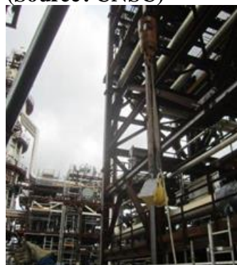
Figure 48: Installation of a fixed gauge by a servicing company (Source: CNSC)
