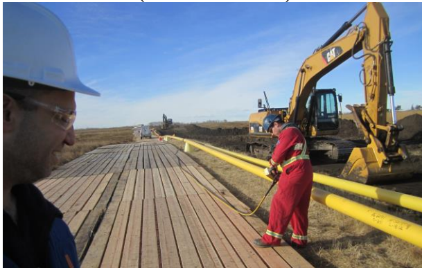
Figure 2: CNSC inspector observes a certified exposure device operator preparing for industrial radiography on a pipeline (Source: CNSC)
