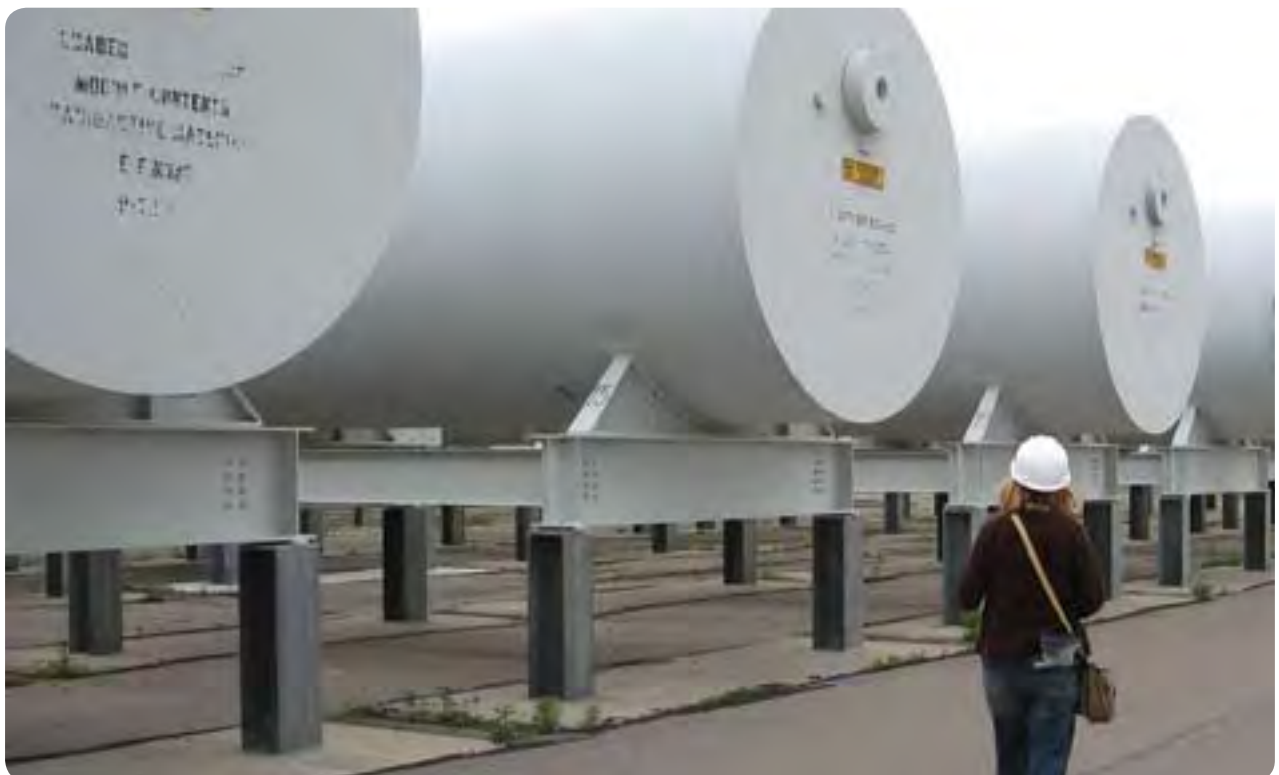
A CNSC Project Officer inspects the re-tube components storage facility at the Pickering Waste Management Facility. The facility stores non-fuel radioactive waste from refurbishment activities at the Pickering Nuclear Generating Station.
