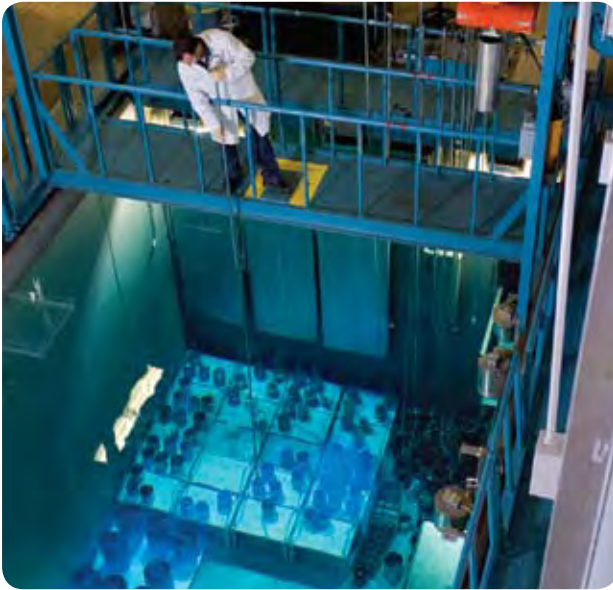
A technician at a CNSC licensee facility inspects the storage of radioactive material in a cooling storage pool.
