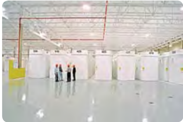
Spent nuclear fuel is placed in secure storage canisters.
