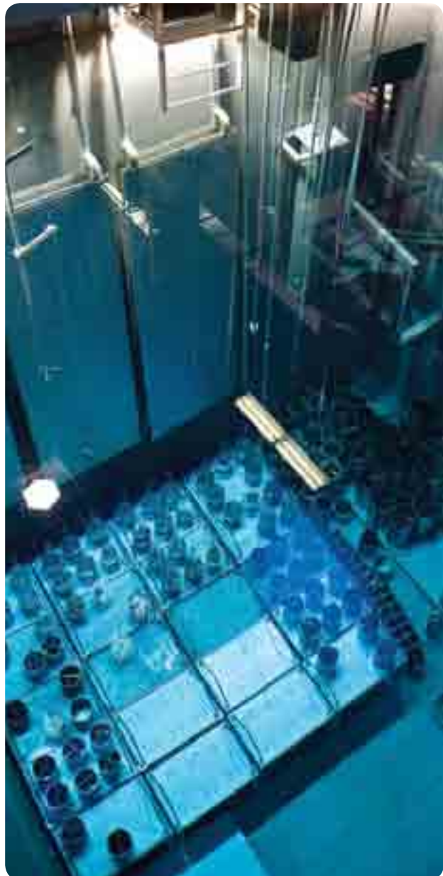
A cooling pool at a CNSC-licensed facility provides safe storage of radioactive material.
