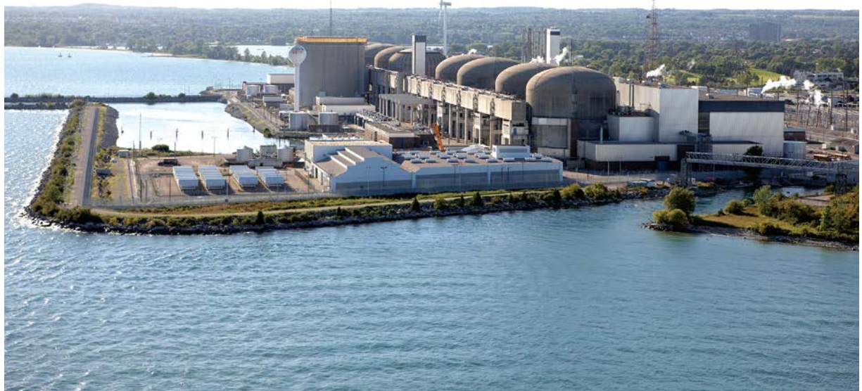
A recent photo of the Pickering Nuclear Generating Station, owned by Ontario Power Generation and located in Pickering, Ontario.
