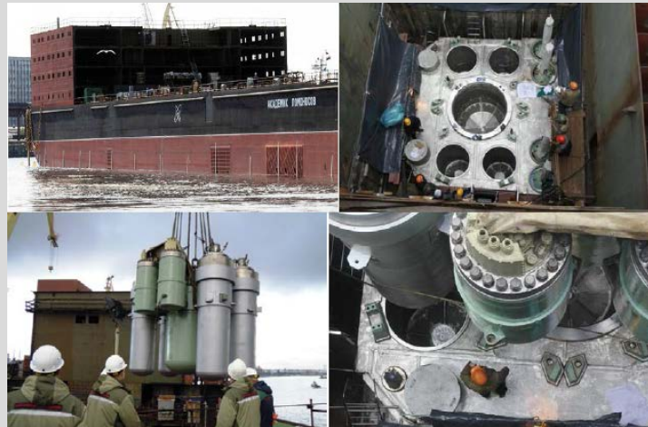
The Russian KLT-40S reactor plant unit being loaded onto a floating nuclear power plant.
