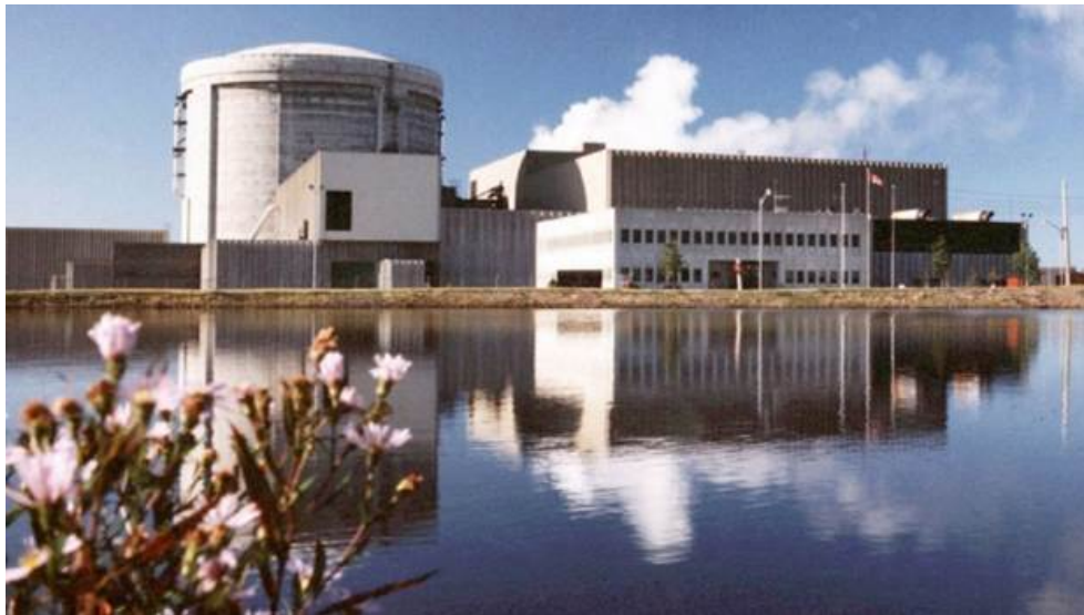
An external view of Point Lepreau Generating Station.
