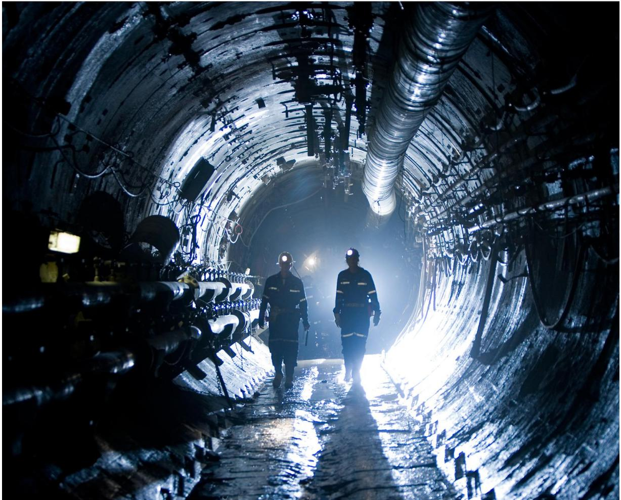
*Underground tunnels at Cigar Lake in northern Saskatchewan.* These tunnels are reinforced with concrete to ensure a safe working environment. The CNSC has full-time staff in Saskatoon and Ottawa who periodically perform inspections to evaluate operations and verify compliance with regulatory requirements and licence conditions.
