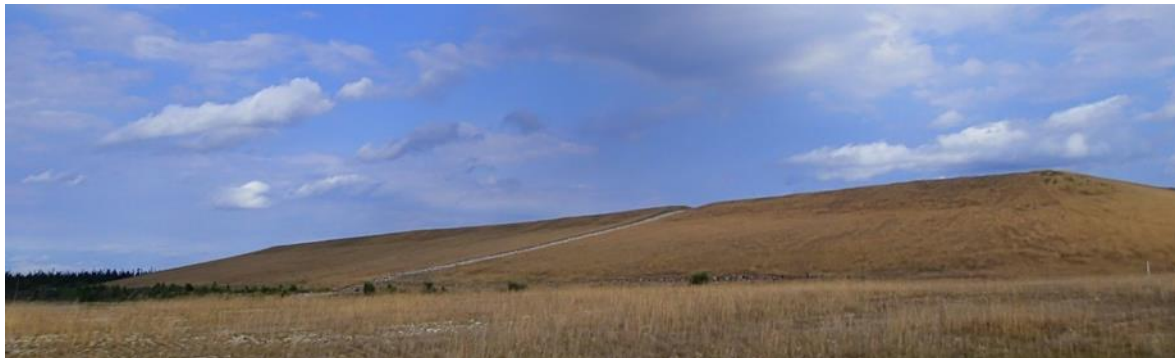
Figure 5-3: Contoured, covered and revegetated B-zone waste rock pile
