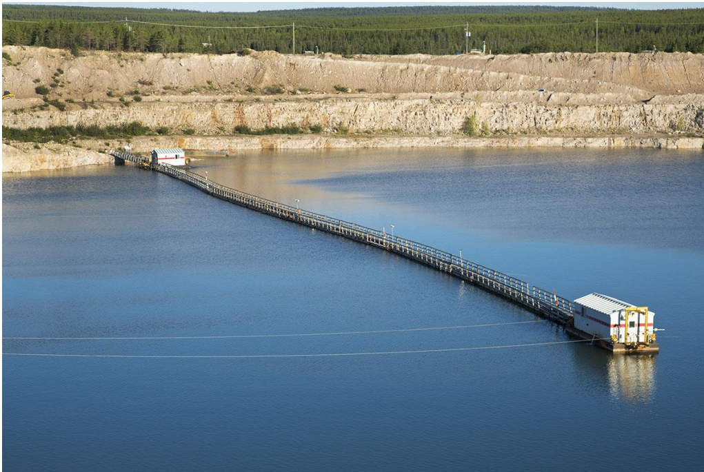
Figure 7-5: McClean Lake operation – JEB tailings management facility
