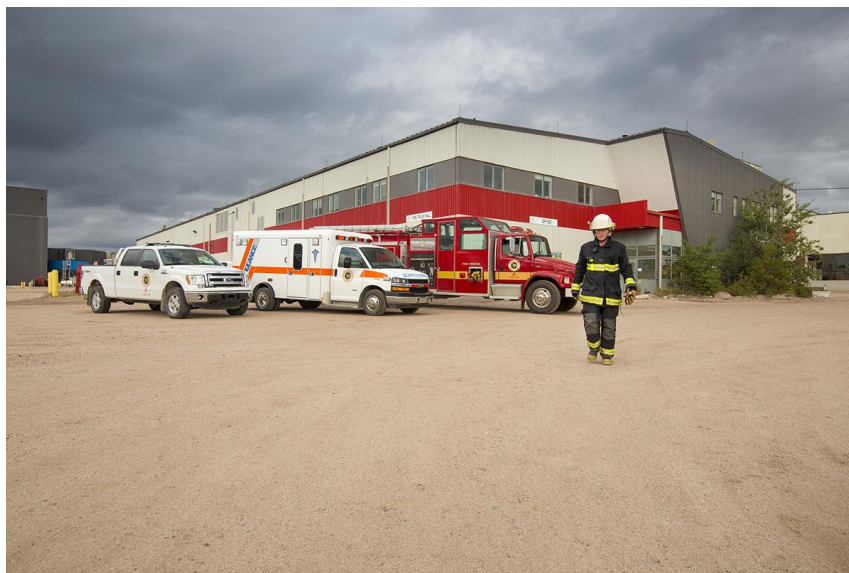
Figure 7-12: McClean Lake operation – emergency response vehicles
