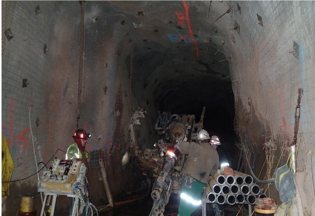
Figure 5-15: Rock bolting and screening observed at Eagle Point work area
