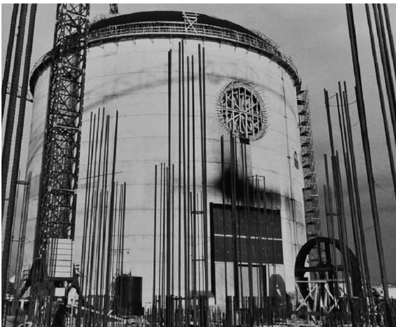
Photo: Construction of Pickering Nuclear Power Station, Ontario.
