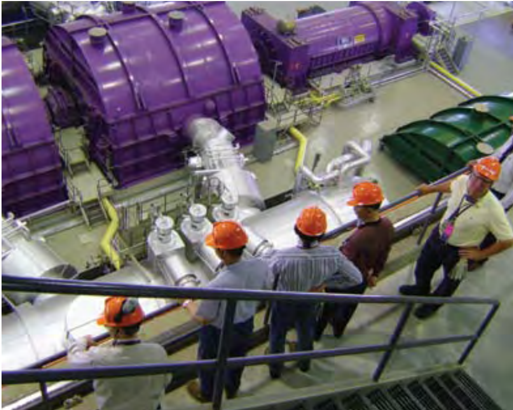
International review team inspectors, accompanied by CNSC staff, overlooking turbine hall at Darlington unit 4.
