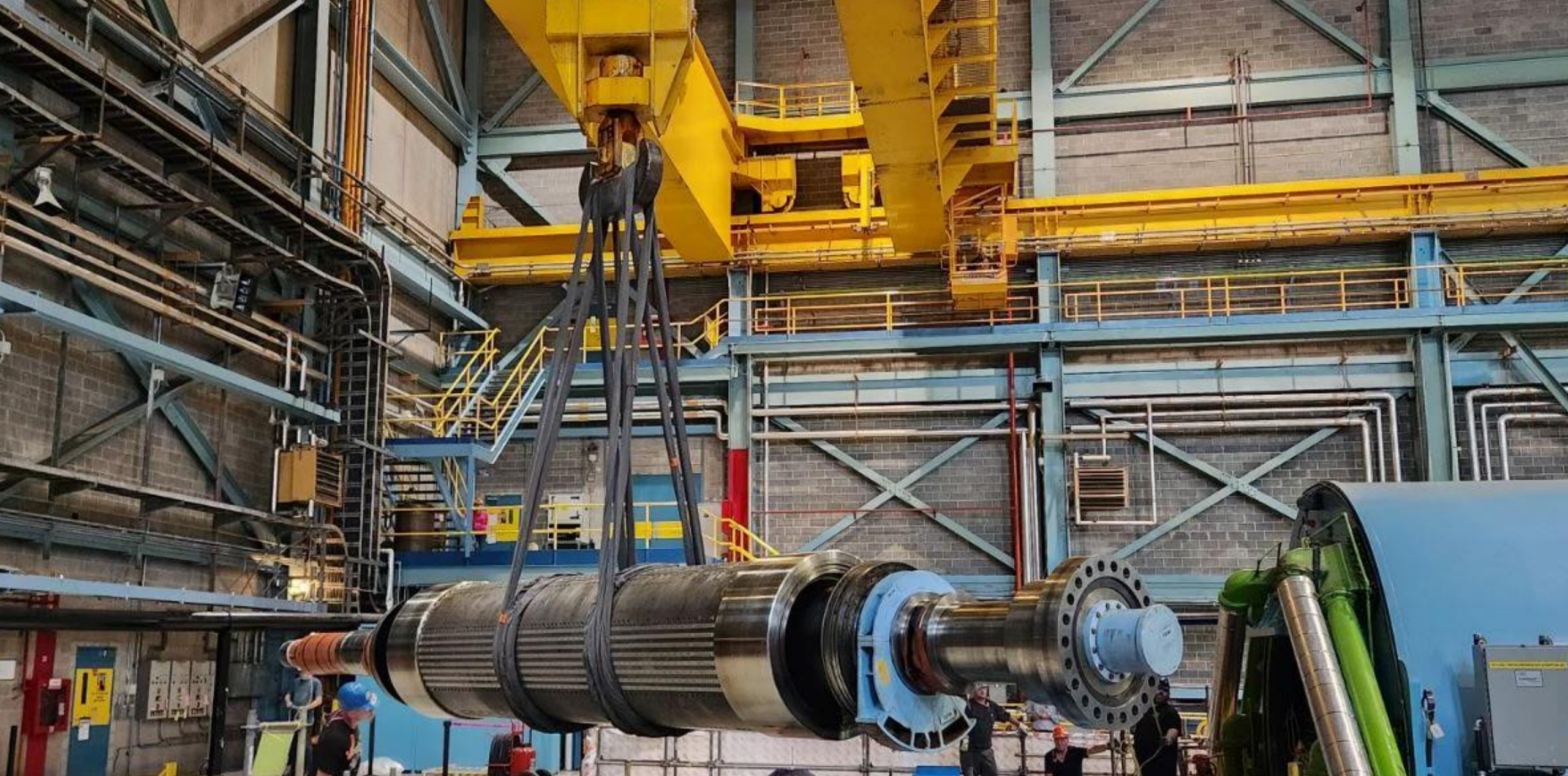
Removal of the Generator Rotor
