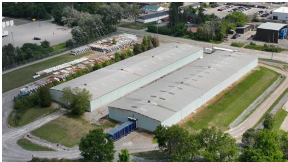
Figure 2 - Site 2, Storage Facility
