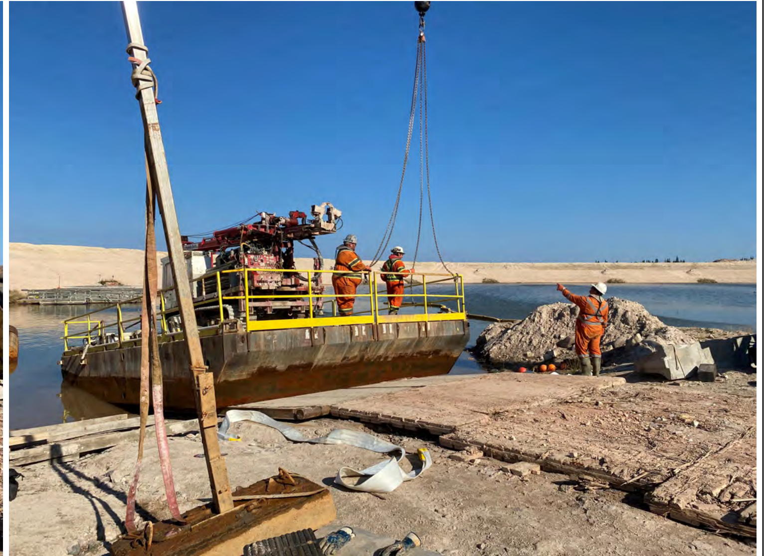
Photo 4: Barge Landing (Part 2)
