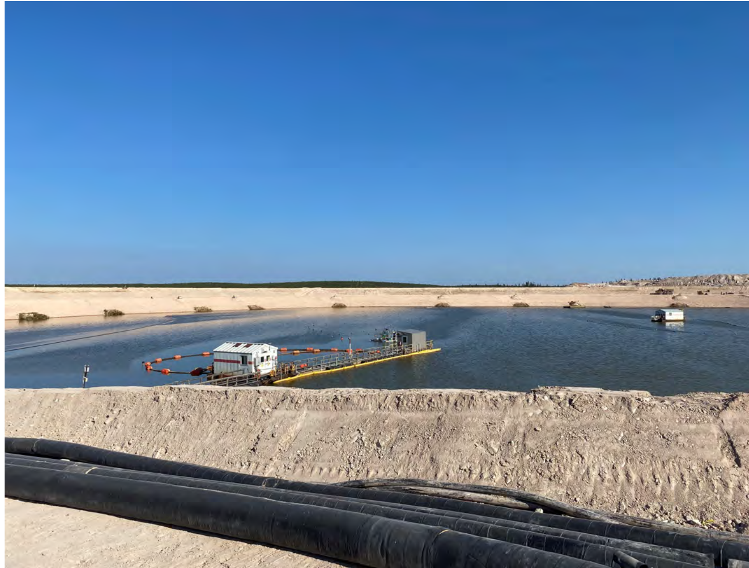
Photo 1: Site overview at the beginning of the day
