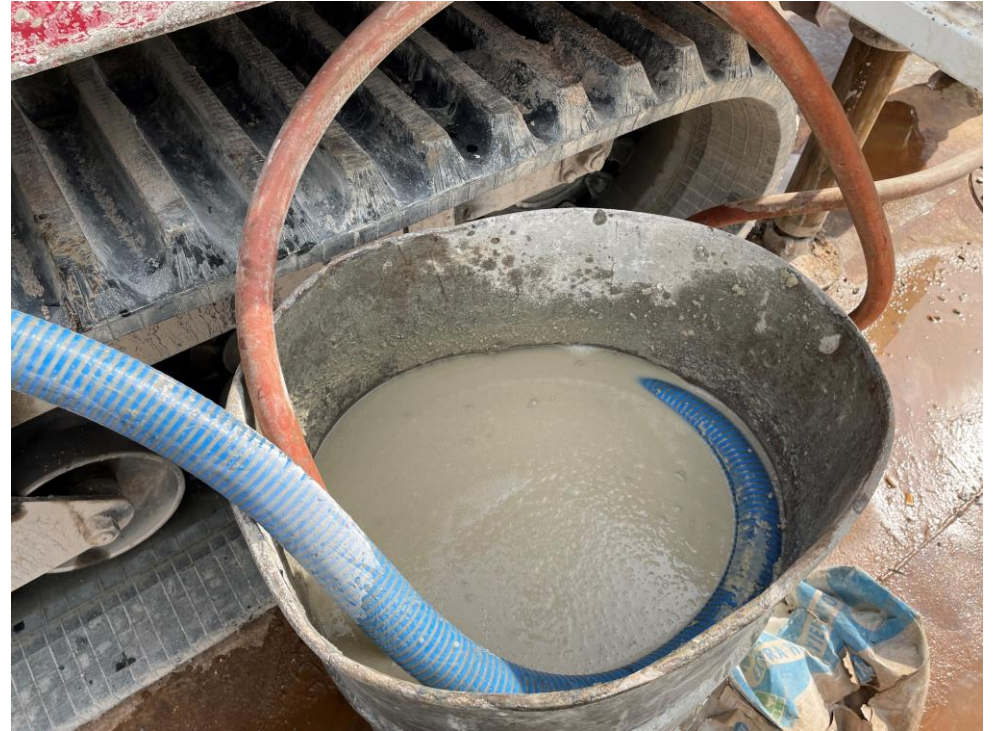
Photo 12: Finished bentonite mixture.
