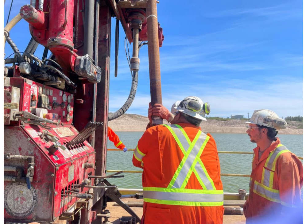
Photo 14: Removal of the casing from TMF24-04.
