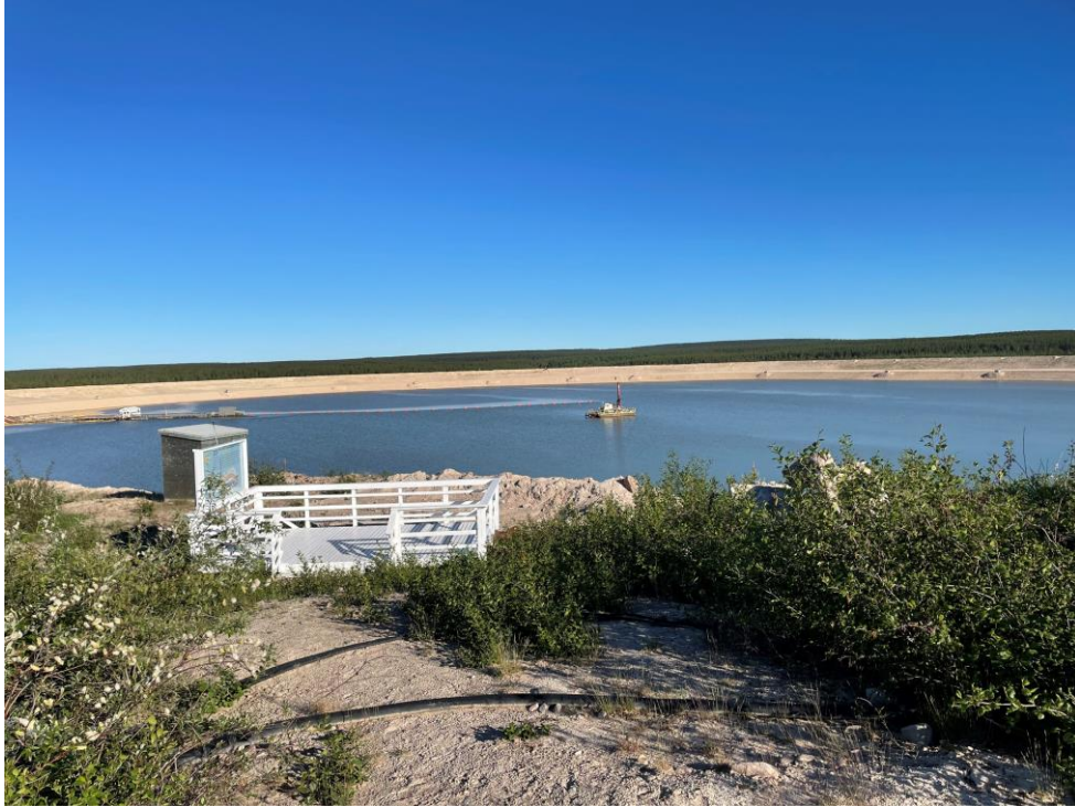
Photo 1: Morning overview of the TMF.
