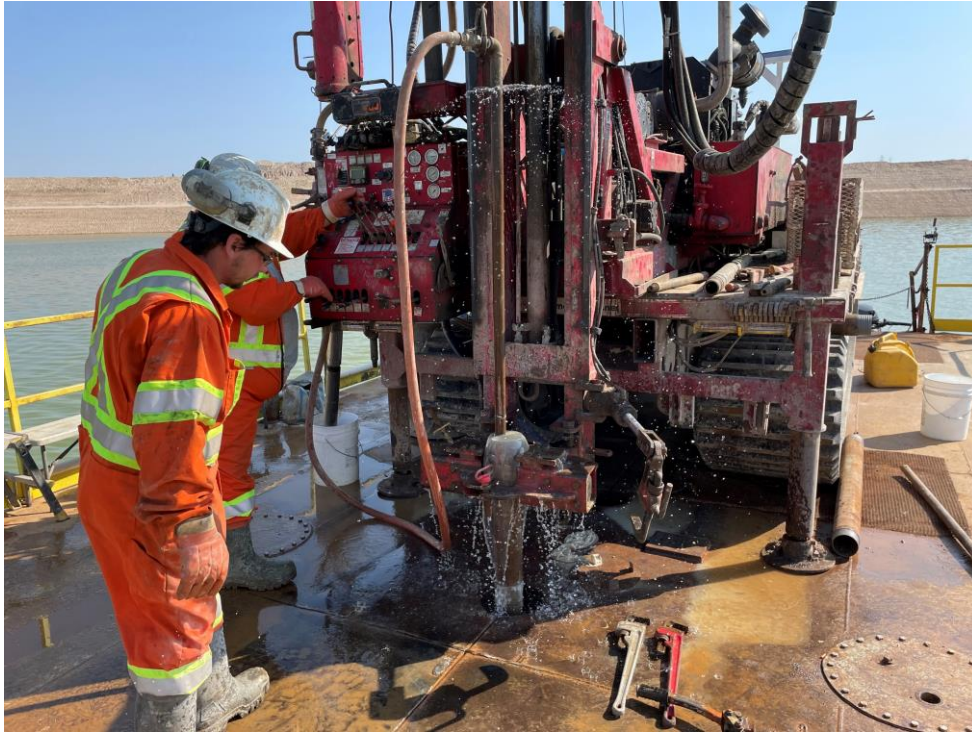
Photo 7: Attempted washing of the casing with a tramline to approximately 0.15 m above target depth.
