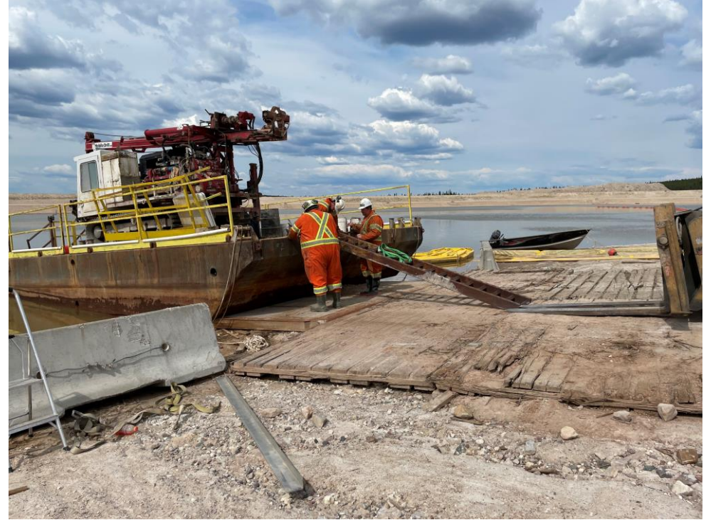
Photo 18: Setting up the tracks to move the drill from the barge.
