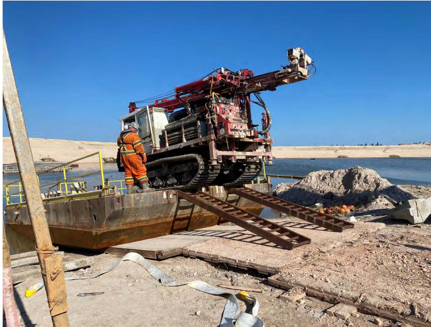
Photo 5: Removal of the Drill from the Barge (Part 1)
