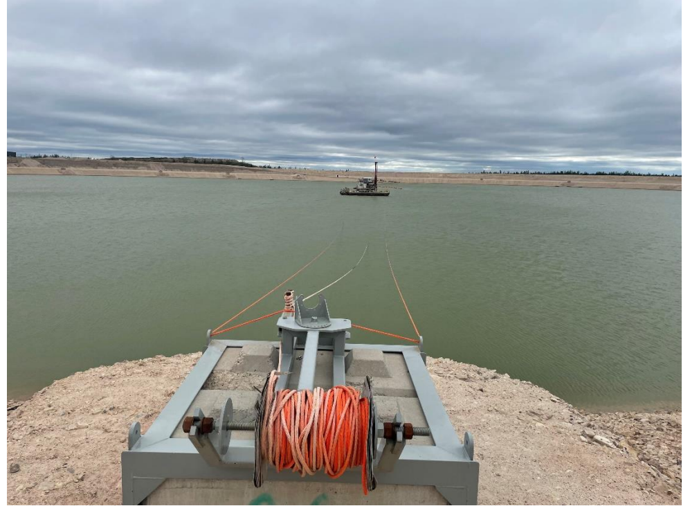
Photo 4: Barge secured to anchor blocks.
