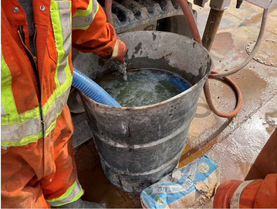
Photo 11: Mixing bentonite with water.
