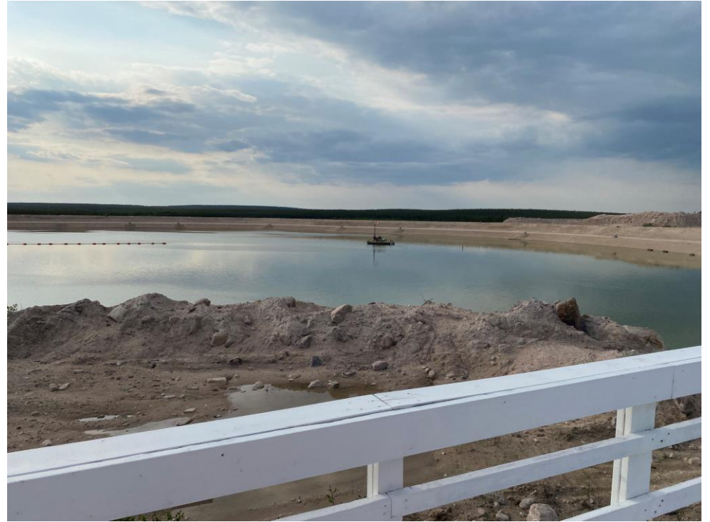
Photo 2: Evening overview of the TMF.
