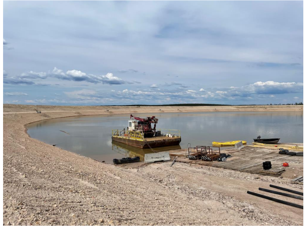
Photo 16: Re-location of the barge closer to the shore.
