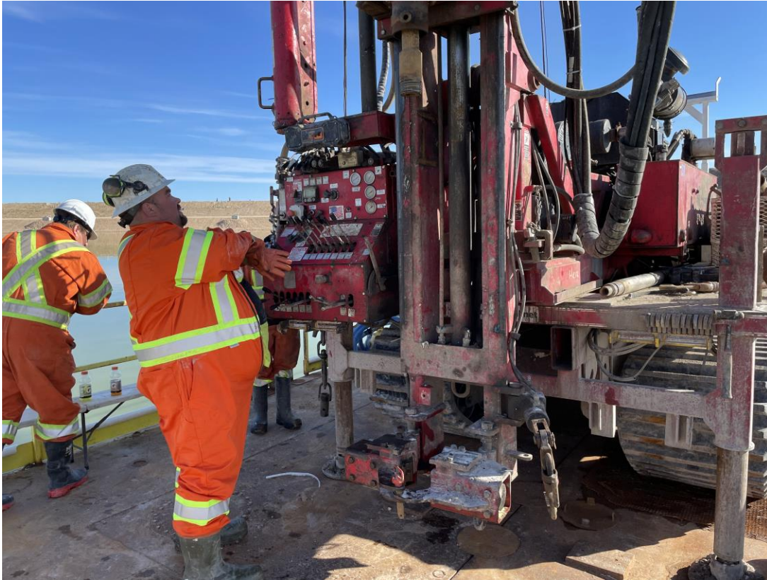
Photo 3: Preparation of the drill before lowering casings into TMF24-04.
