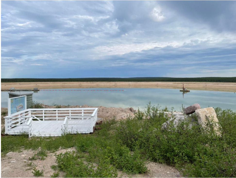
Photo 1: Morning overview of the TMF.
