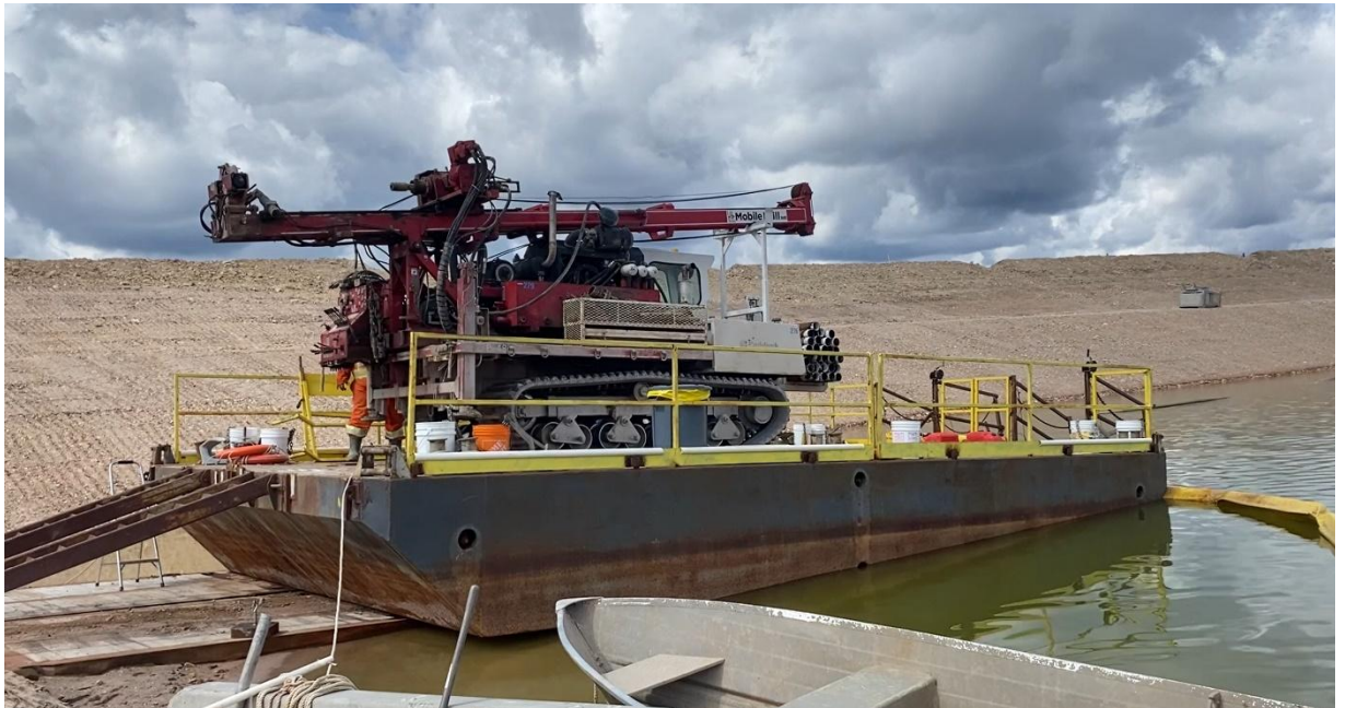
Figure 1: Barge and Drill Rig Set-Up
