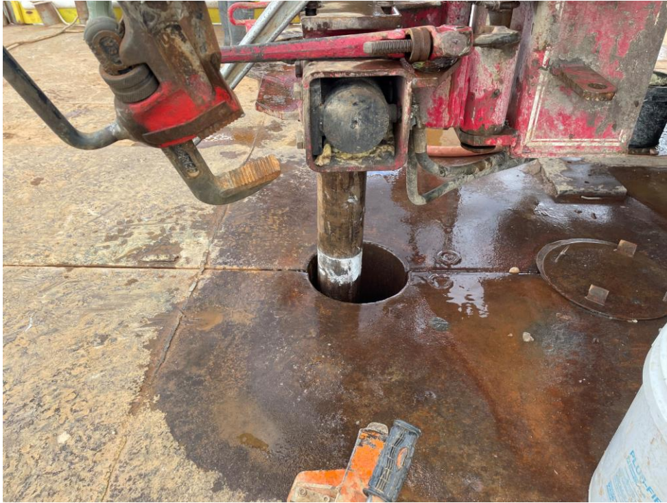
Photo 16: The drill casing angled under the barge as increasing wind gusts became present.
