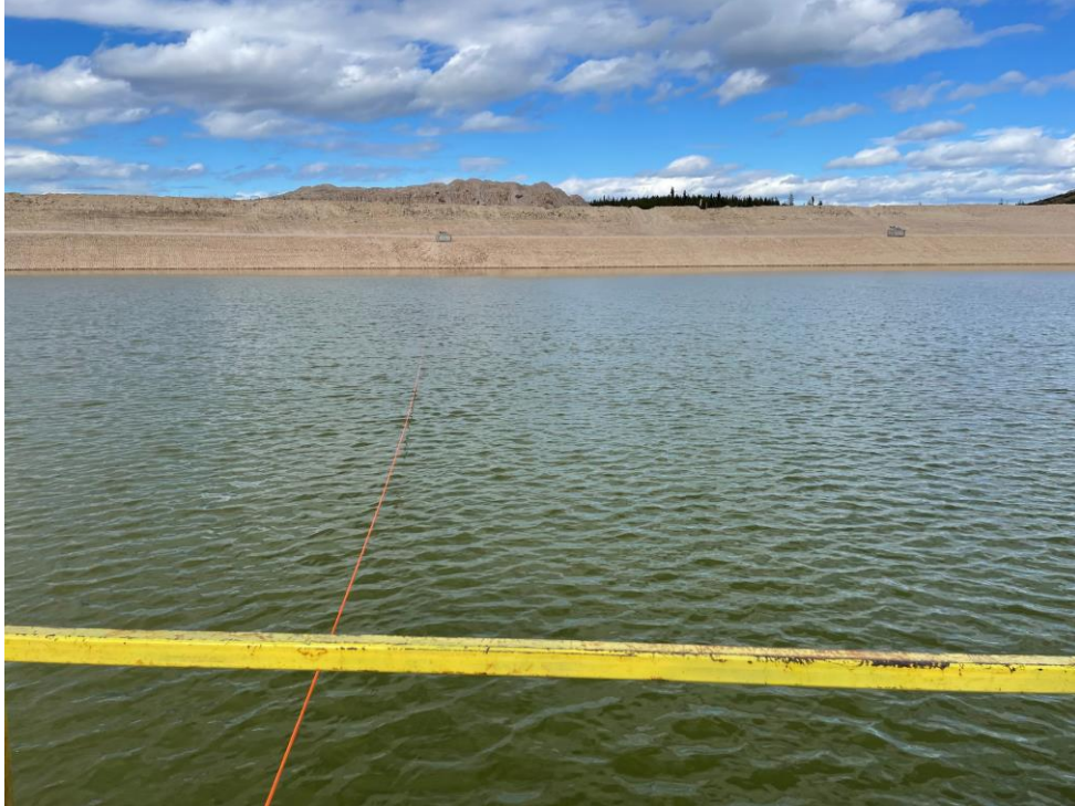
Photo 29: Attachment of the barge to the block anchor during relocations to counteract the wind gusts
