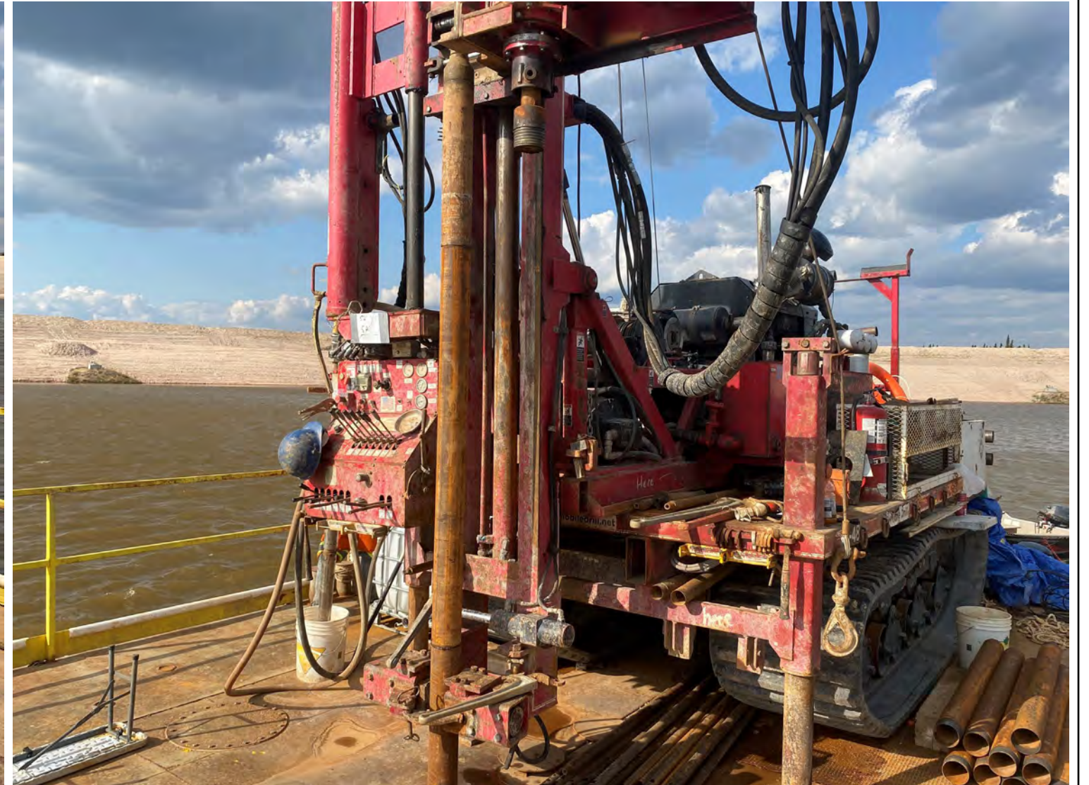
Photo 4: Steel Casing Corner View
