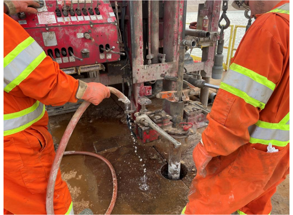
Photo 2: Pushing the first Shelby tube (TMF24-14-SA01A).
