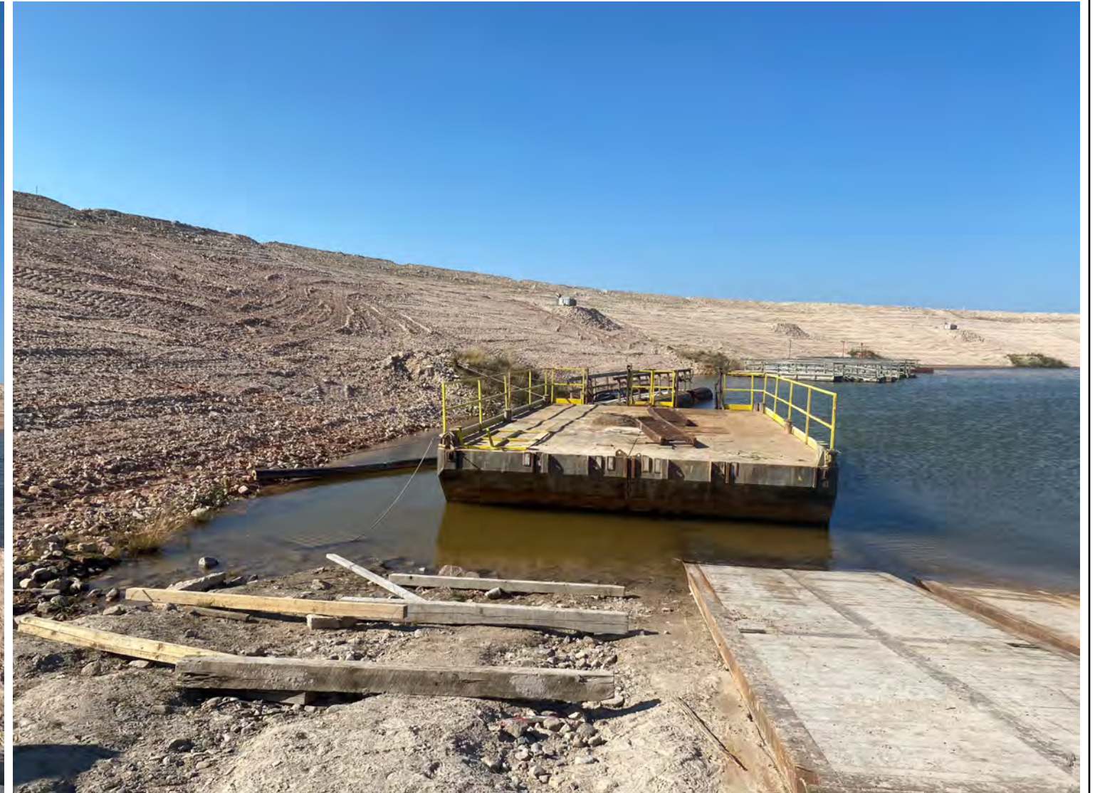
Photo 2: Barge location in the afternoon
