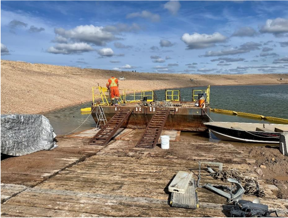
Photo 3: Preparation of the barge for drill loading.
