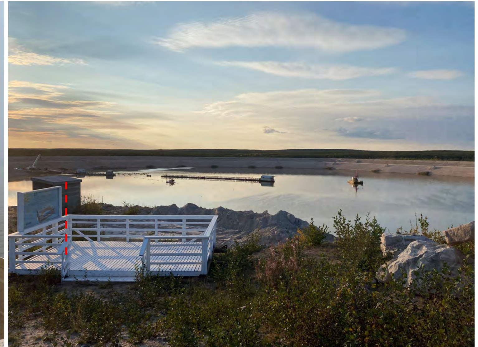
Photo 2: Site overview at the end of the day
