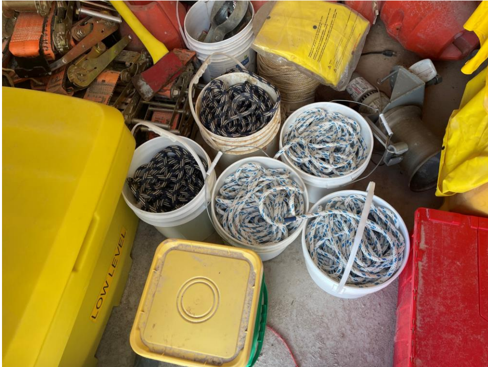
Photo 4: New anchor ropes prepared for drilling tomorrow.
