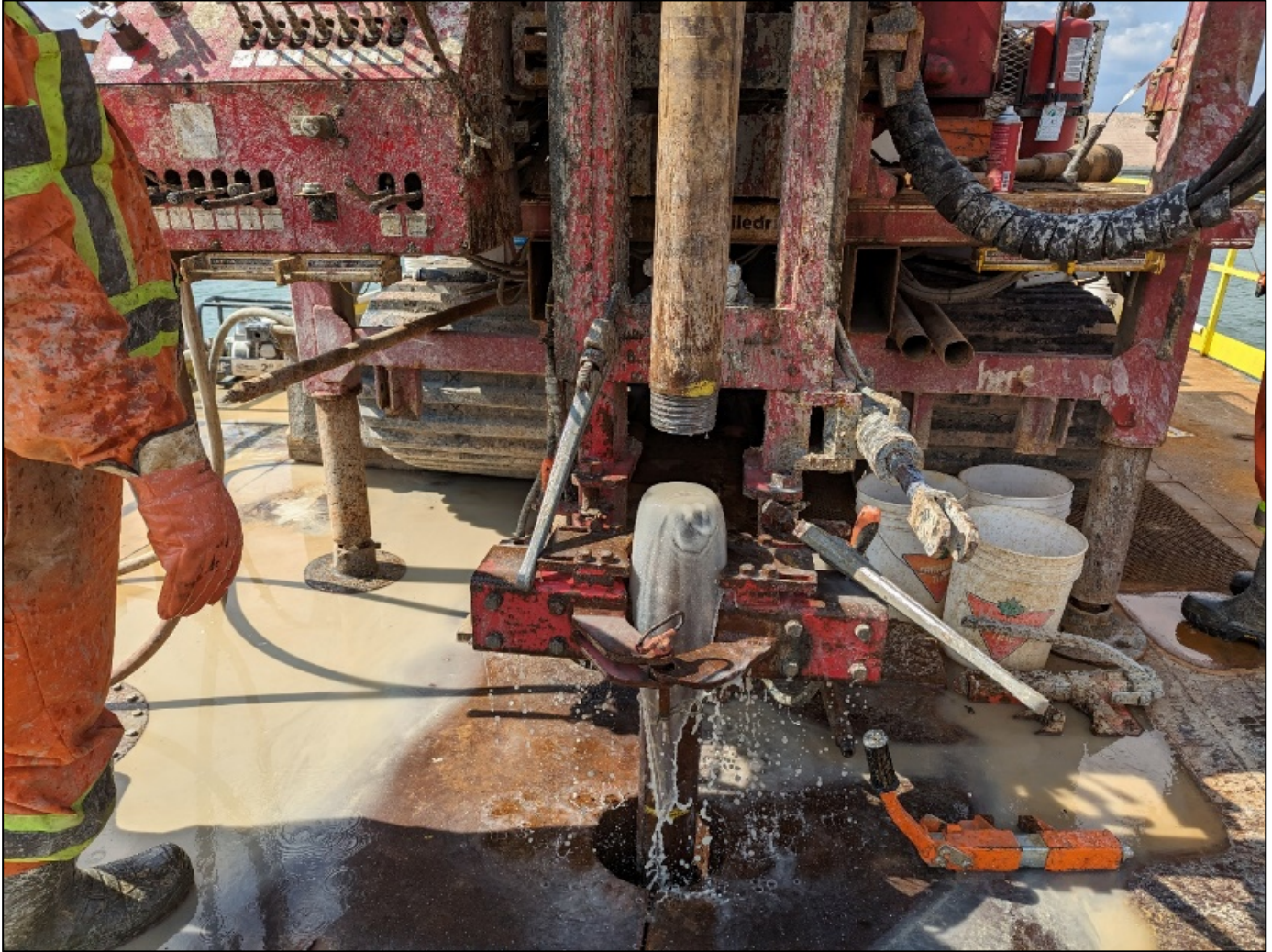
Figure 5.6-19: A "jet" of water observed at surface after stopping casing advancement. Note that the artesian flow was temporary and typically stopped within a couple minutes.
