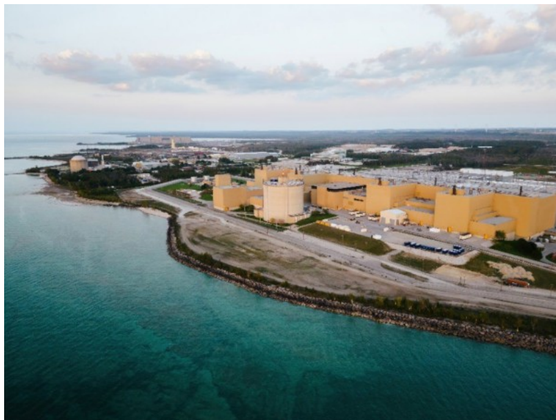
Figure 1. Bruce B Nuclear Generating Station (Image Courtesy of Bruce Power).
