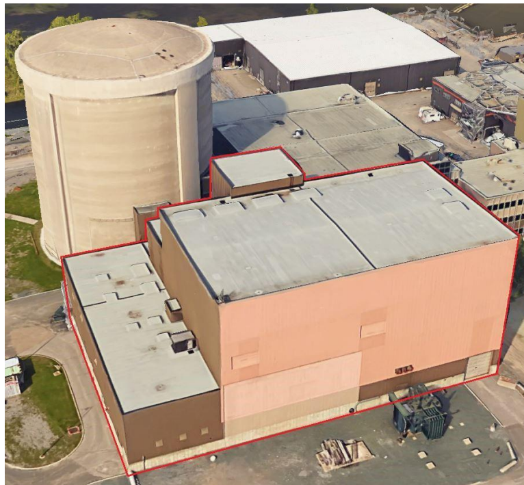
Figure 4 : Turbine Building (bordered by red markings)
