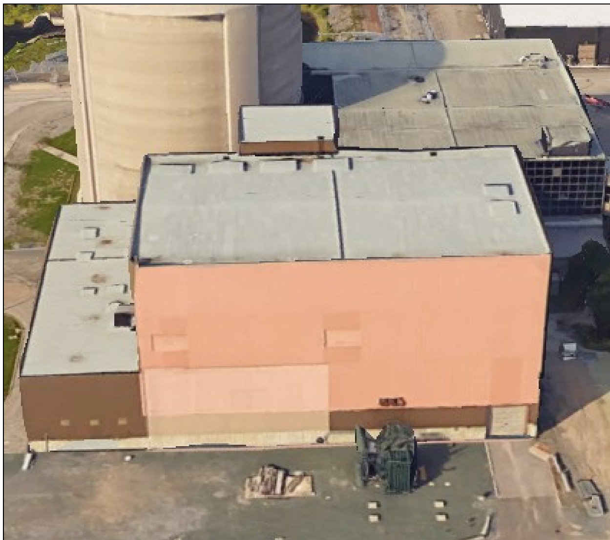
Figure 12: Turbine Building Exterior View (Eastward)
