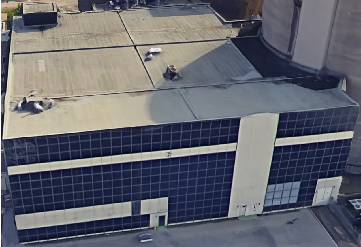
Figure 10: Service Building Exterior View (Southward)
