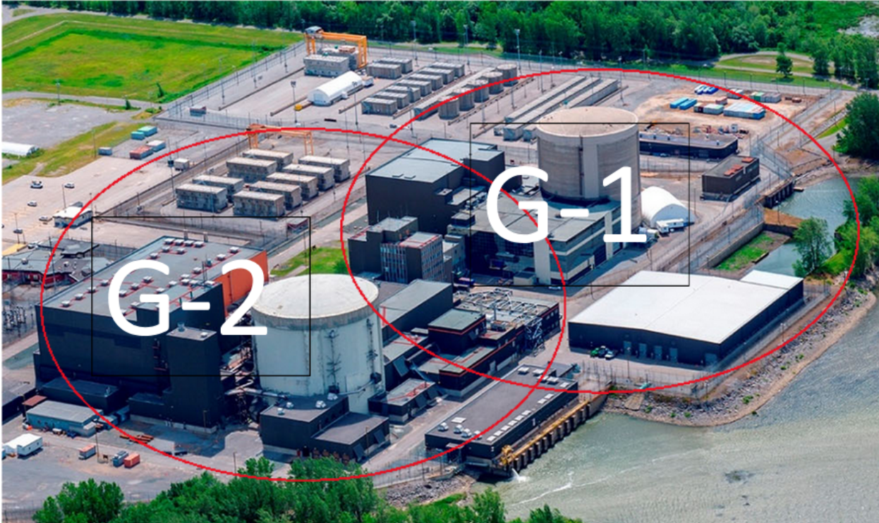
Figure 1. The Gentilly site, comprising the Gentilly-1 and Gentilly-2 Waste Facilities, is on the south shore of the St. Lawrence River in Bécancour, Québec.
