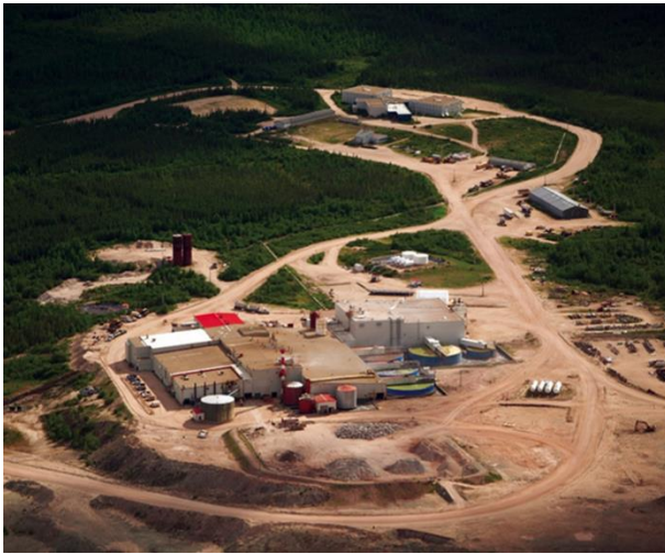
Figure 3.3.1: Rabbit Lake Operation – mill aerial view
