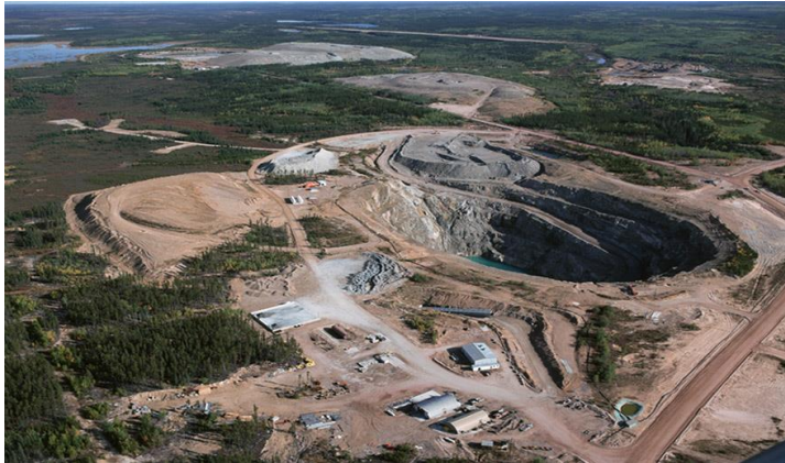
Figure 8.3.1: Cluff Lake Project – pre-decommissioning view, 2009
