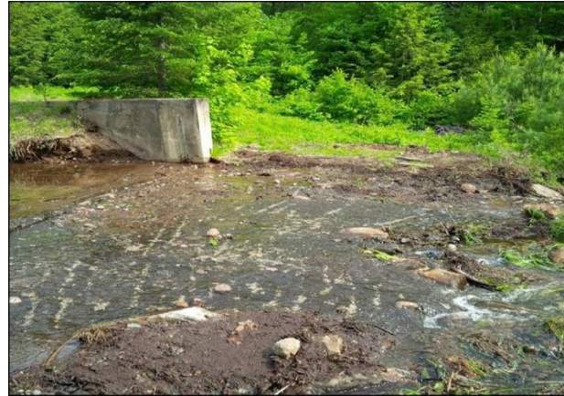
Figure 8.7.1: Bicroft – spillway of Pond A at the tailings management facility, 2017
