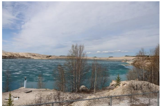
Figure 3.4.2: Deilmann tailings management facility
