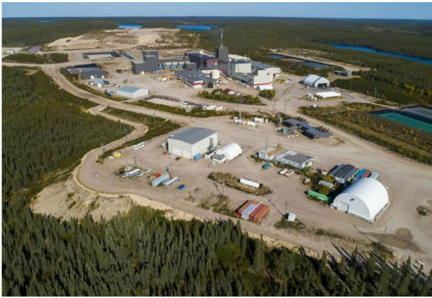
Figure 3.5.1: McClean Lake Operation – aerial view
