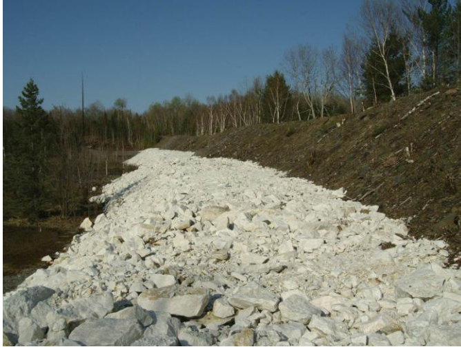
Figure 8.8.1: Dyno – dam and toe berm
