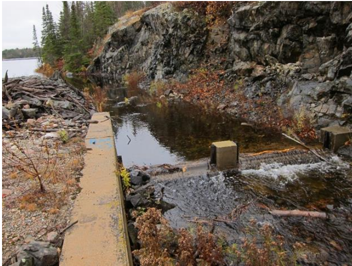
Figure 8.9.1: Elliot Lake – spillway at the Quirke mine site
