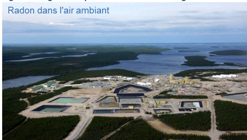
Figure 3.1: Cigar Lake Operation - aerial view looking north
