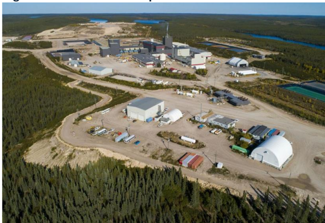
Figure 3.5 McClean Lake Operation - aerial view
