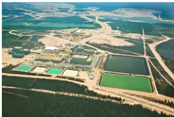
Figure 3.4 Key Lake Operation - aerial view
