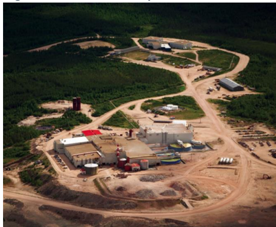
Figure 3.3: Rabbit Lake Operation - aerial view of Mill
