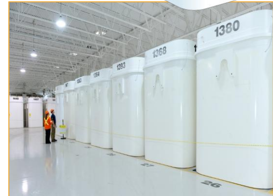
OPG Used Fuel DSCs stored at the Western Waste Management Facility
