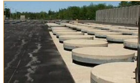
Darlington Storage Overpacks for ILW from refurbishment located at the Darlington Waste Management Facility
