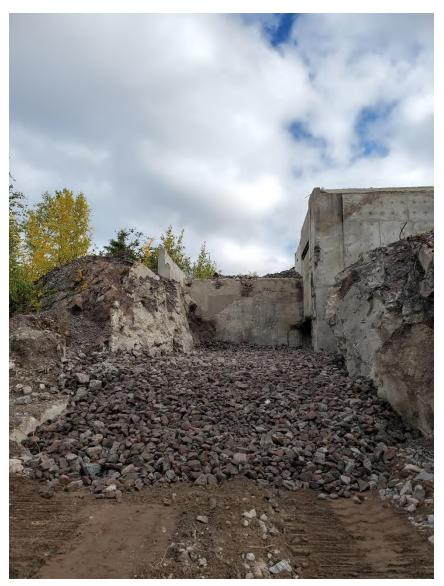
Photo 17: Additional placement of coarse waste rock over Raise 3 and 2, up to the entrance at Raise 1.
