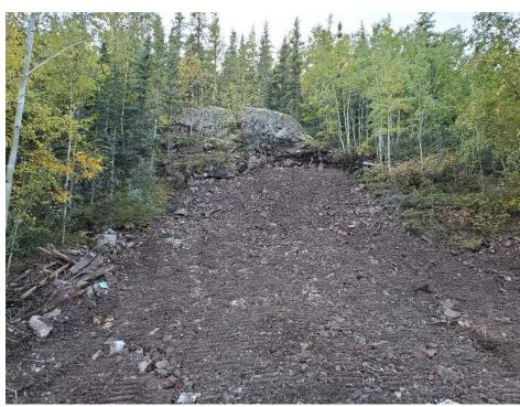
Photo 5: Final Placement of Backfill material along the Fishhook Bay Adit.
