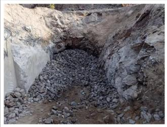
Photo 8: Placement of sorted waste rock (competent rock passing approximately 200 mm).
