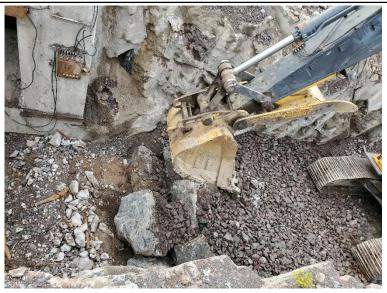
Photo 12: Placement of coarse waste rock over the boulders at Raise 3 to safely access Raise 2.
