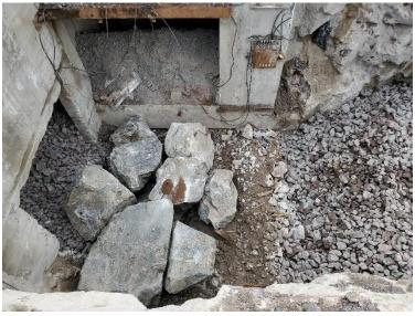
Photo 15: Top view of the 11 boulders placed at Raise 2.
