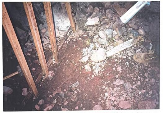
Photograph 3: Debris removed approximately 2 ft. to rock and backfilled on completion at bottom end.
