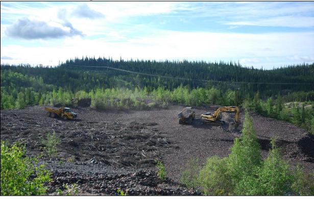
Figure 5: Sorted Waste Rock Used for Backfill Material
