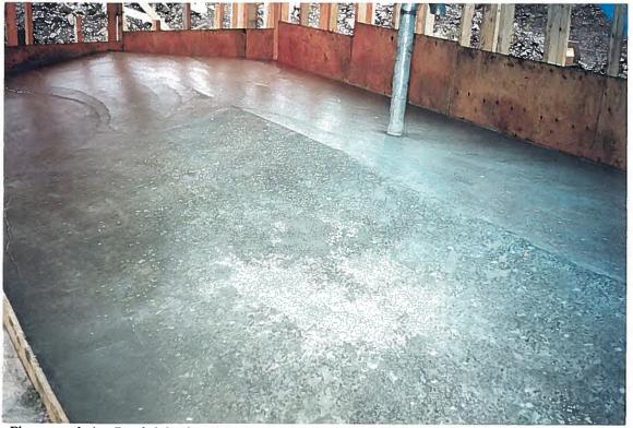
Photograph 6: Roof slab after the steel trowel finish.
