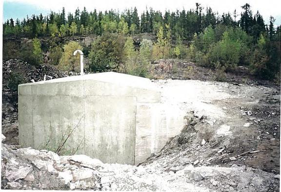
Photograph 7: Completed structure after the forms were removed.
