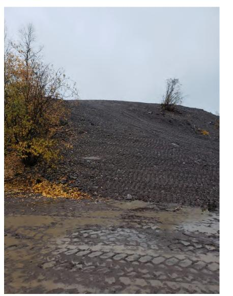
Photo 19: Final placement of the gravel cover layer.
