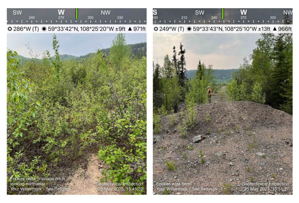
Photo C6 – View of vegetation establishing along drainage channel (May 2023).
