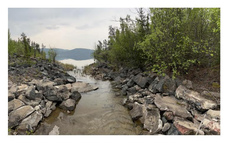
Photo B5 – Fookes Reservoir Spillway showing broken rip-rap on north and south sides of channel. Note debris has been removed since 2022 inspection.
