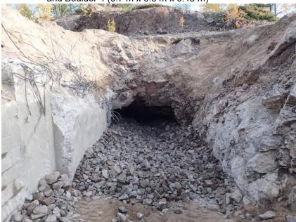
Photo 7: Placement of sorted waste rock (competent rock passing approximately 200 mm)
