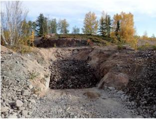
Photo 9: Placement of sorted waste rock, tight against the back (competent rock passing approximately 200 mm).
