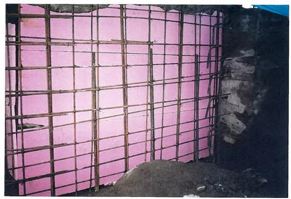
Photograph 3: Form break and rebar on the walls. Note: the rebar detail was revised to tie into existing wall.
