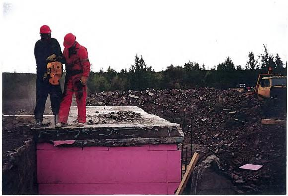
Photograph 2: Demolition of the existing ridge cap.
