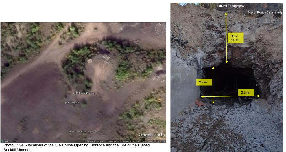
Photo 2: Overview of the CB-1 Mine Opening and Dimensions. Cables and conveyer belt visible within the opening.
