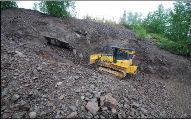
Figure 7: Placing Sorted Waste Rock in Adit Entrance
