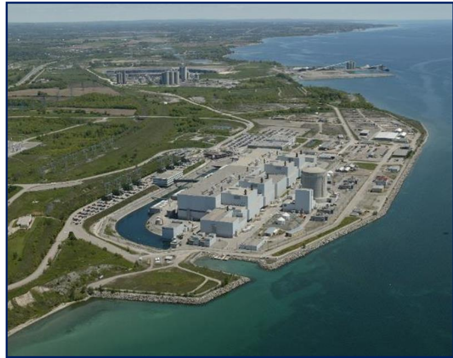
Darlington Nuclear Generating Station. Source: OPG
