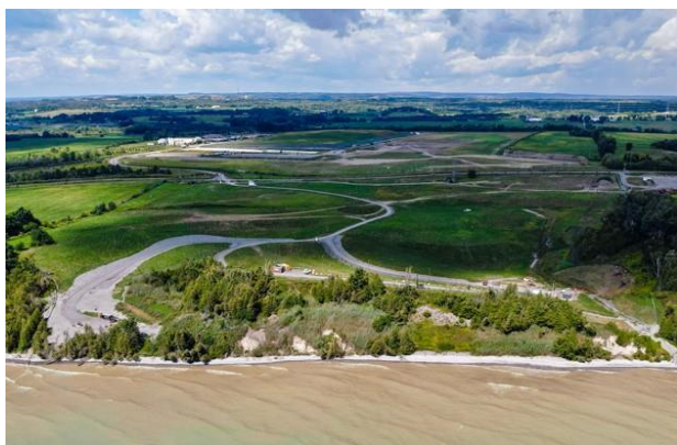
Figure 5: Port Granby – Remediation Completed (Source: CNL)
