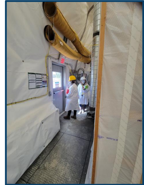
CNSC staff performing an inspection at Whiteshell Laboratories. Source: CNSC staff
