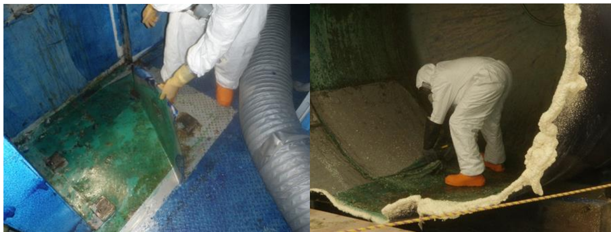
Figure 17: Application of decontamination strippable gel during Building 200 decommissioning.
