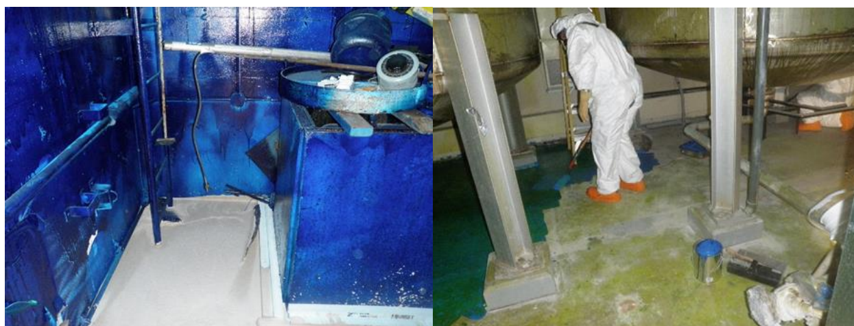
Figure 18: Grouting and fixatives for Building 200 demolition.
