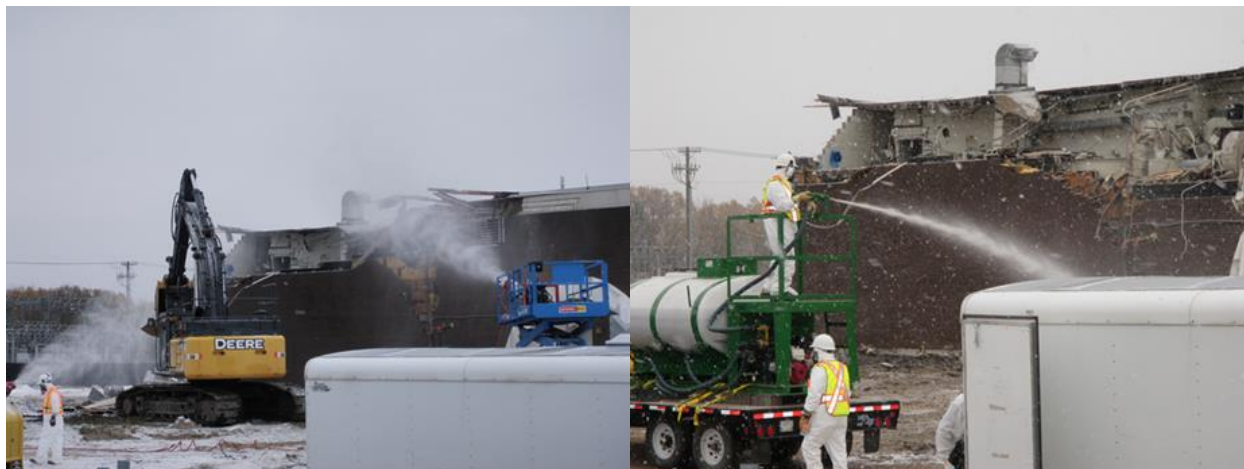
Figure 19: Application of water misting and a fixative agent during Building 200 open air demolition.
