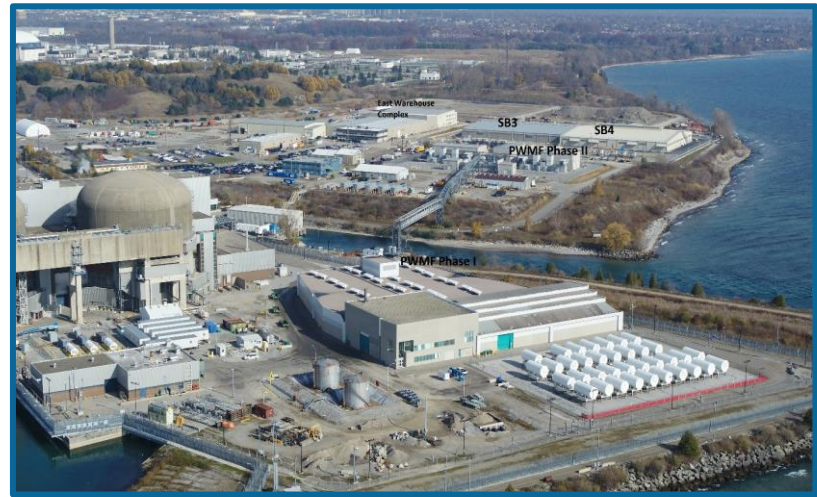
Aerial view of Pickering Waste Management Facility Source: OPG
