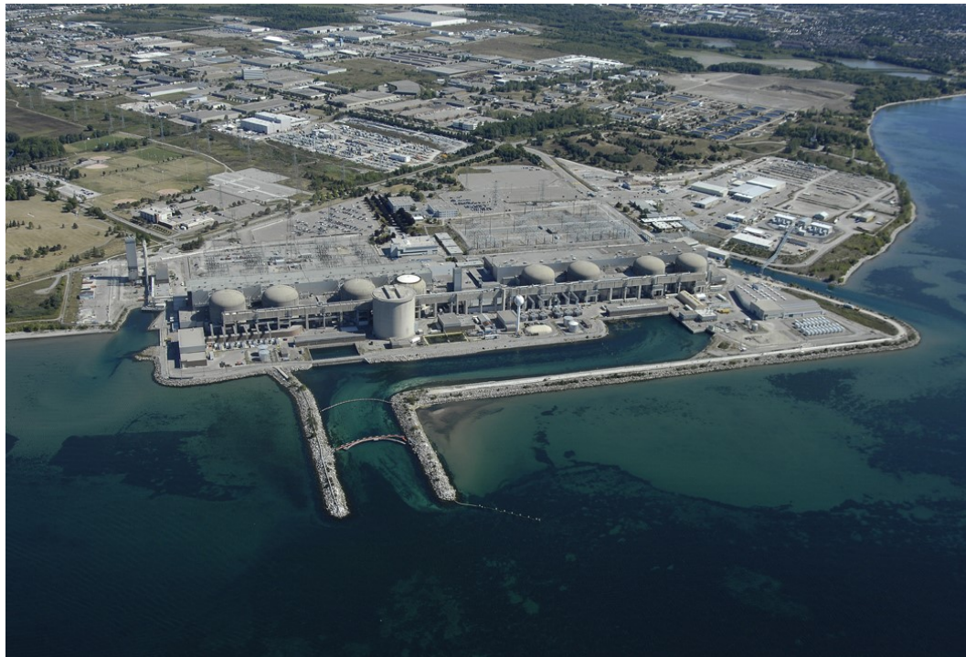
Figure 1- Pickering Nuclear Generating Station
