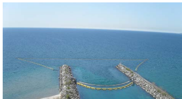
FIGURE 38 - FISH DIVERSION SYSTEM
