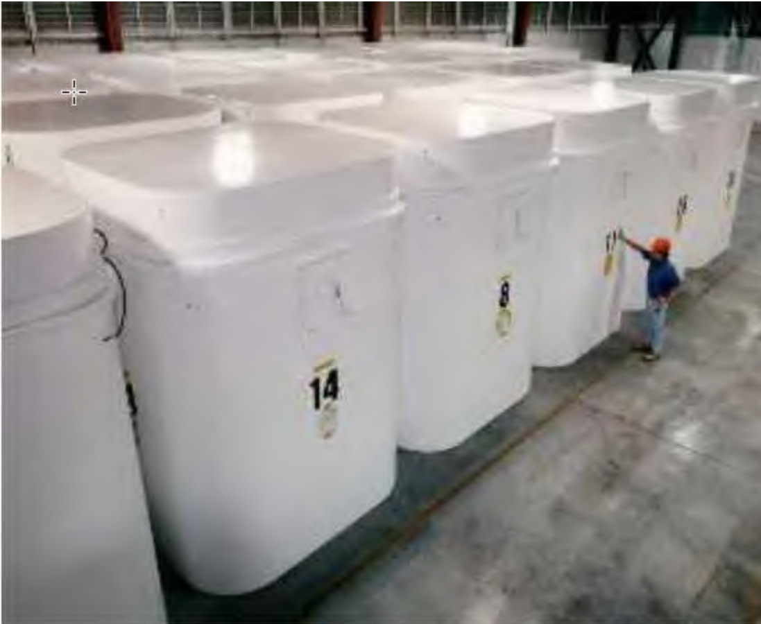
Figure 4-5: Typical DSC Storage at PWMF
