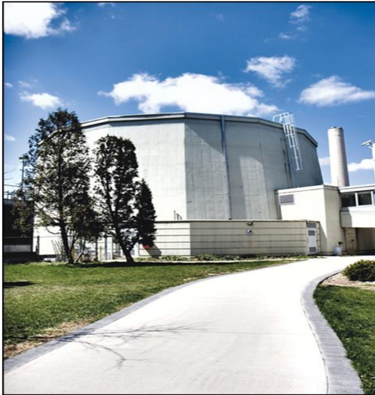
Figure 1-2: McMaster Nuclear Reactor
