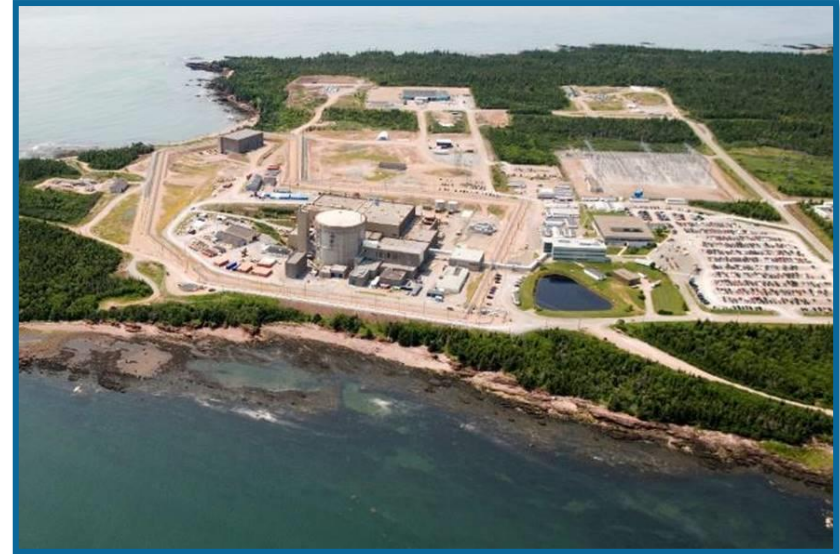
Point Lepreau Nuclear Generating Station Source: NB Power
