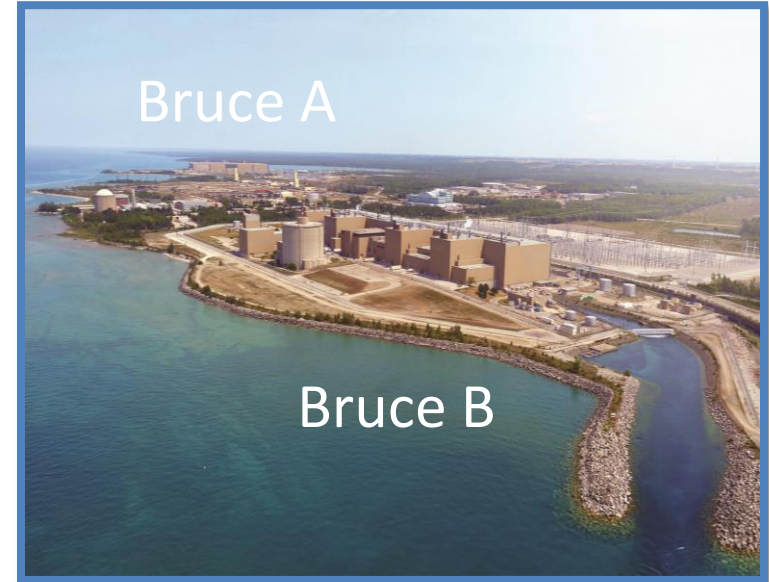
Bruce A and Bruce B Nuclear Generating Stations Source: Bruce Power
