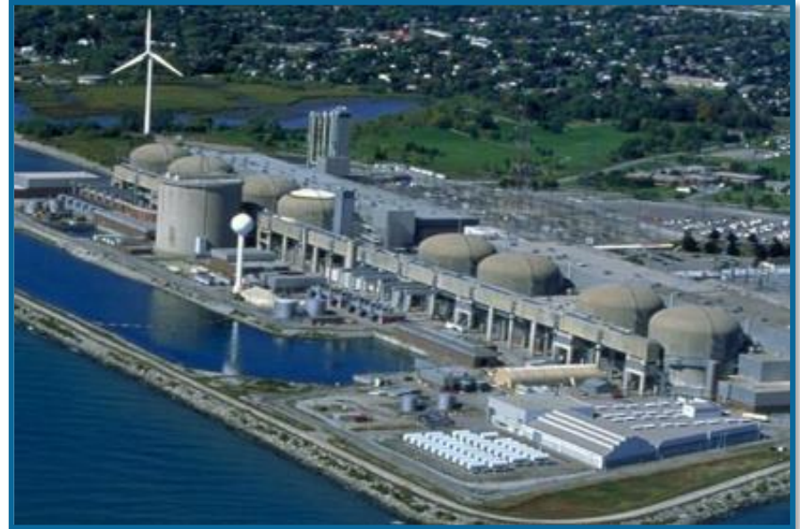
Pickering Nuclear Generating Station
