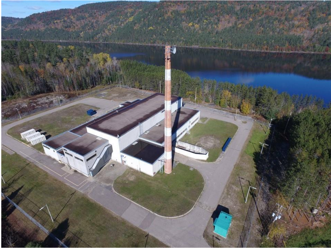
Figure 8: Nuclear Power Demonstration Waste Facility (Source: CNL)
