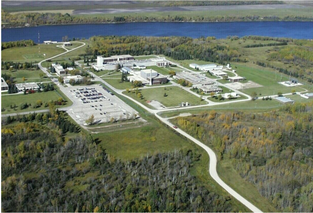
Figure 3: Whiteshell Laboratories main campus (Source: CNL)
