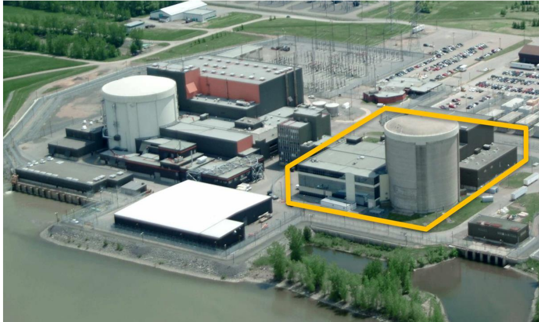
Figure 7: Gentilly-1 Waste Facility, outlined in yellow (Source: CNL)
