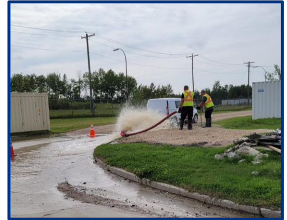
Flow test of fire hydrant. Source: CNSC staff
