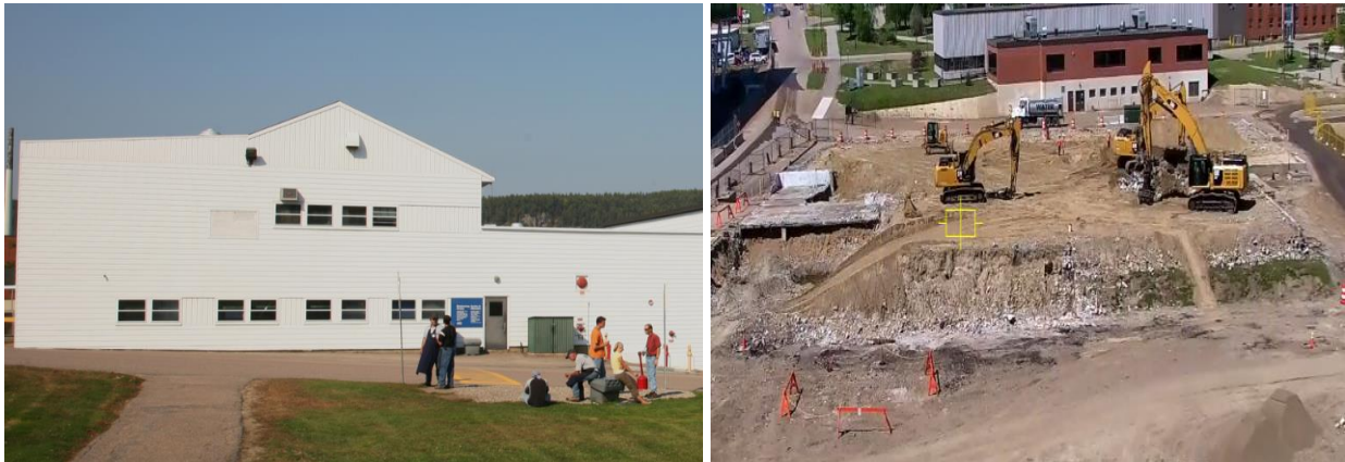
Figure 26: Machine, Welding, and Sheet Metal Shops and Administration Services – Before, After
