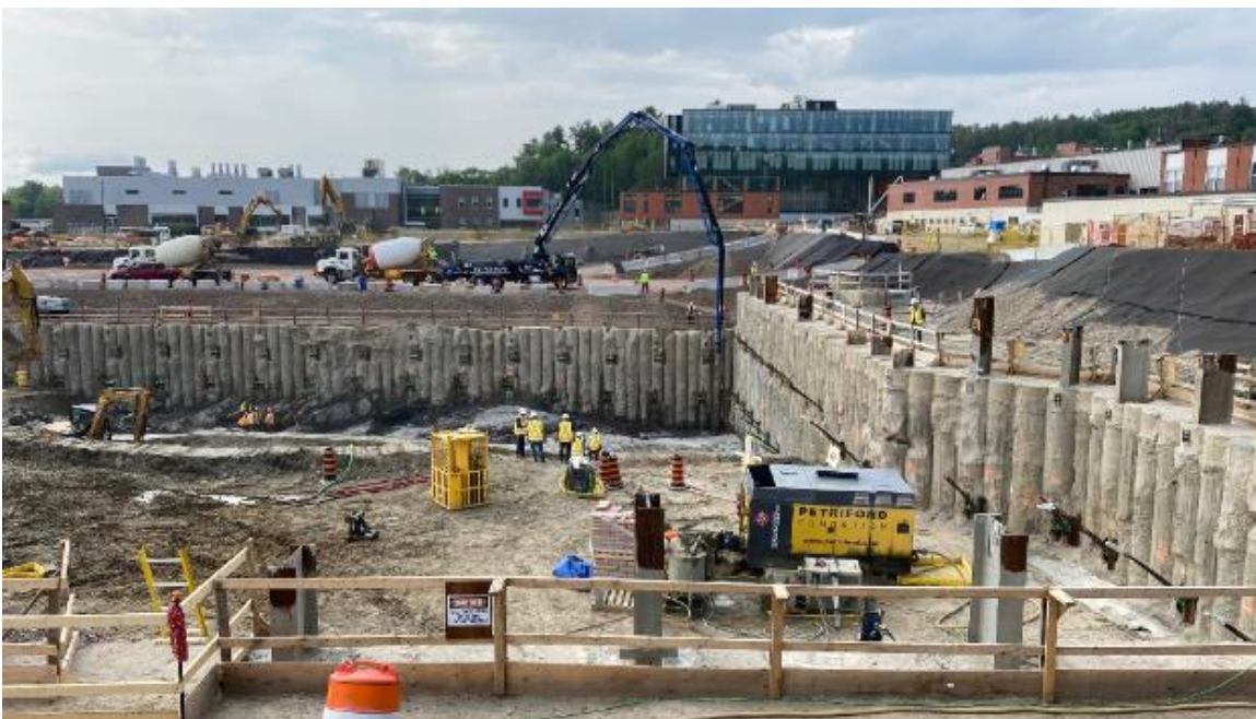
Figure 16: Sub-foundation of the Advanced Nuclear Materials Research Centre
