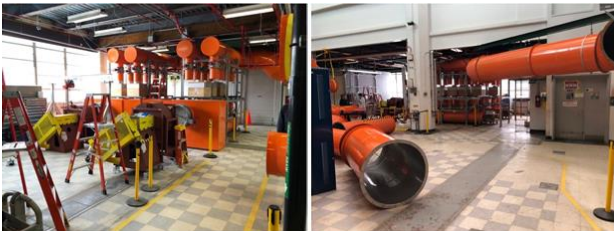
Figure 40: Replacement of the Reactor Ventilation System
