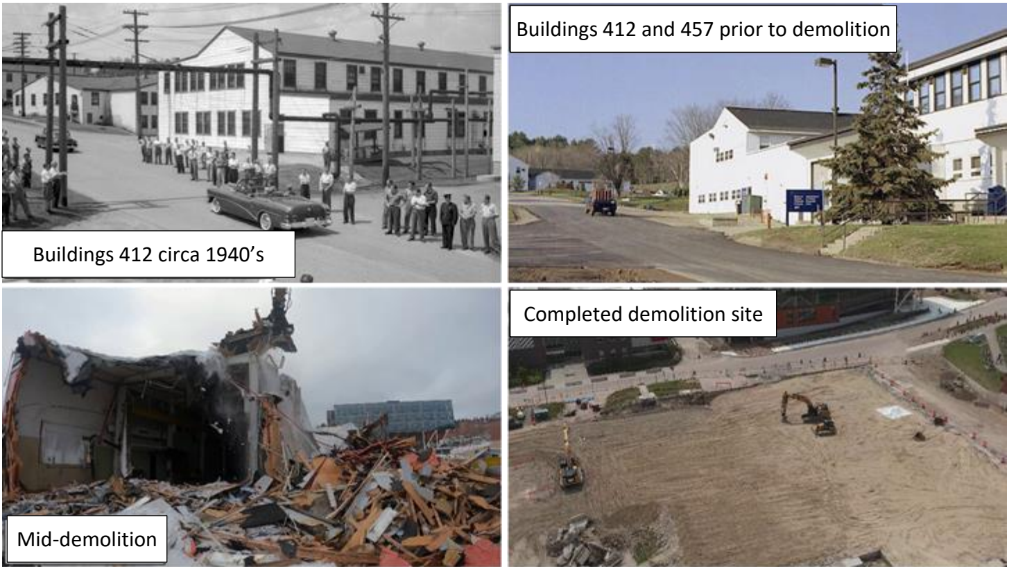
Figure 30: Demolition of Buildings 412 and 457
