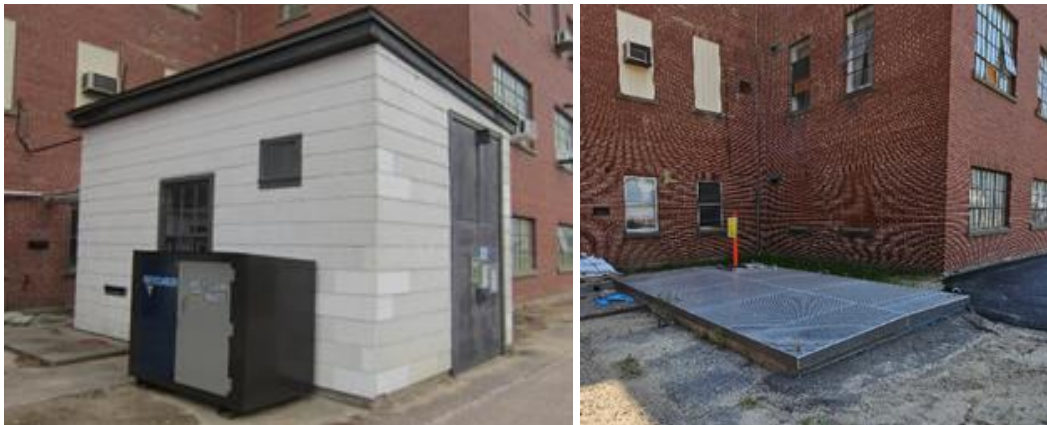
Figure 24: National Research Experimental Reactor Effluent Experimental Building – Before, After
