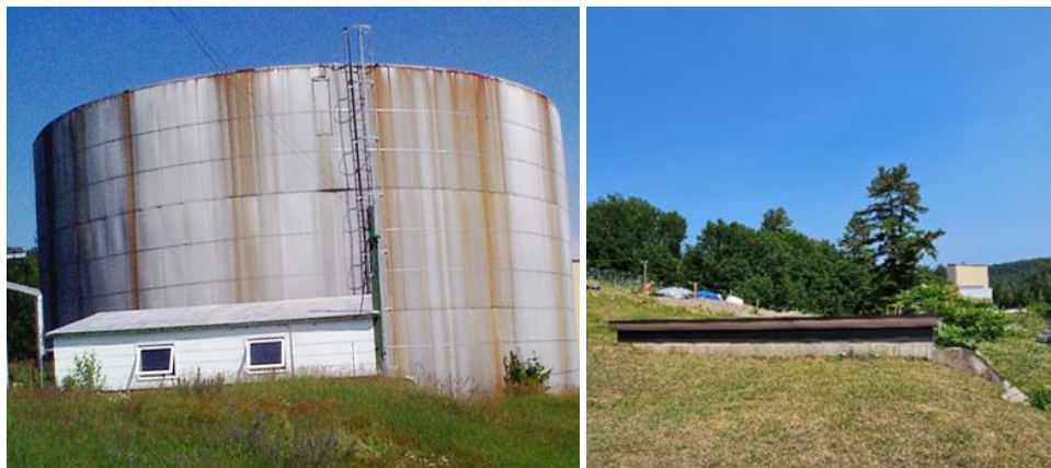
Figure 27: Former Filtered Water Storage Reserve – Before, After
