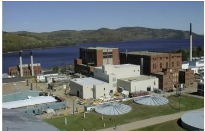
Figure 29: Facilities to be Decommissioned
