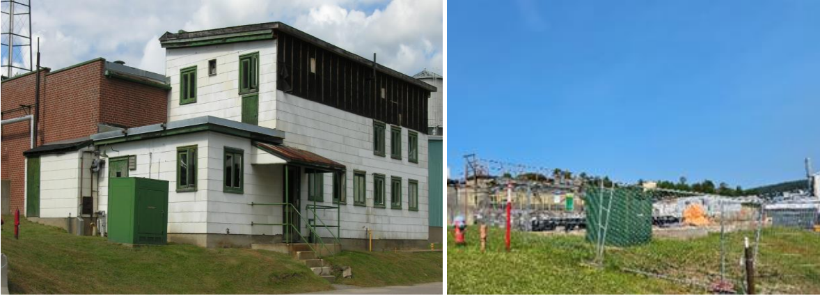
Figure 25: Mixed Waste Storage – Former Heavy Water and Drum Cleaning Building / Former Change House – Before, After
