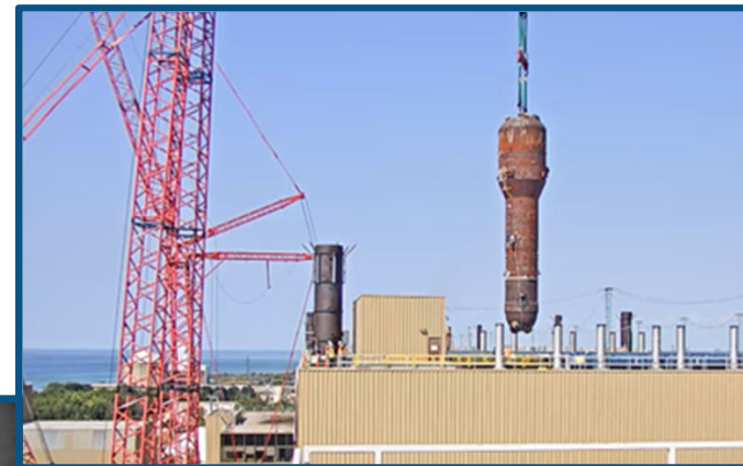
Left: Steam generator being removed
