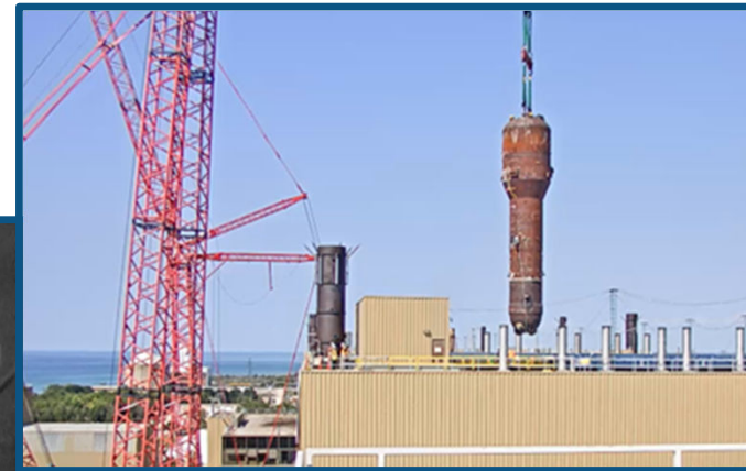
Left: Steam generator being removed Bottom: Fuel channel installation activities
