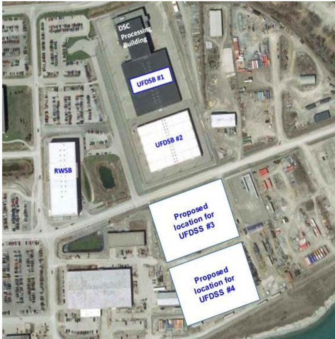
Figure 1: Darlington Waste Management Facility (DWMF)
