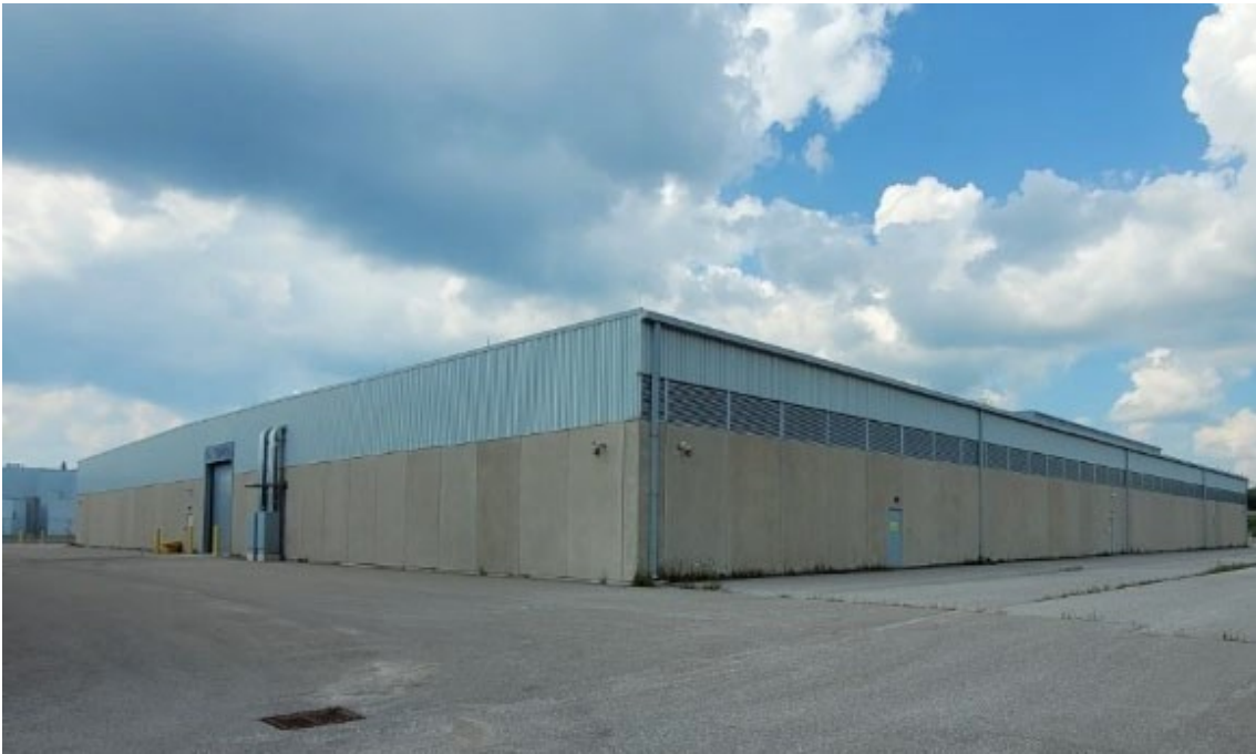
Figure 4: Used fuel Dry Storage Building #1
