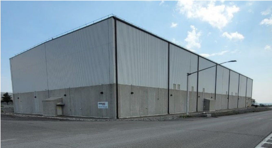
Figure 6: Retube Waste Storage Building
